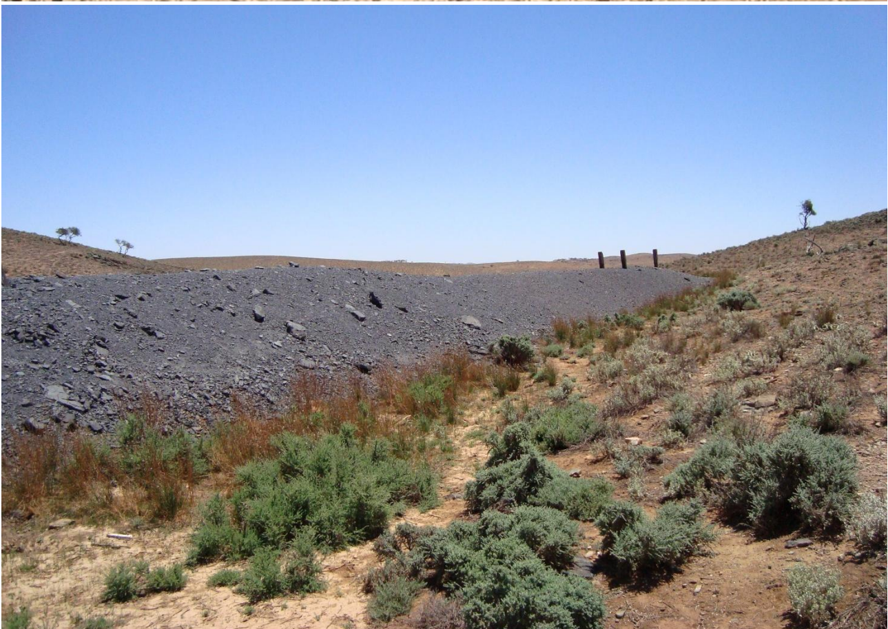
Plate 3-9: Adit and residual stockpile, Razorback
