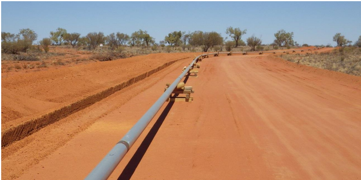
Plate 4-1: Buried flowline prior to being laid in the trench during construction.
