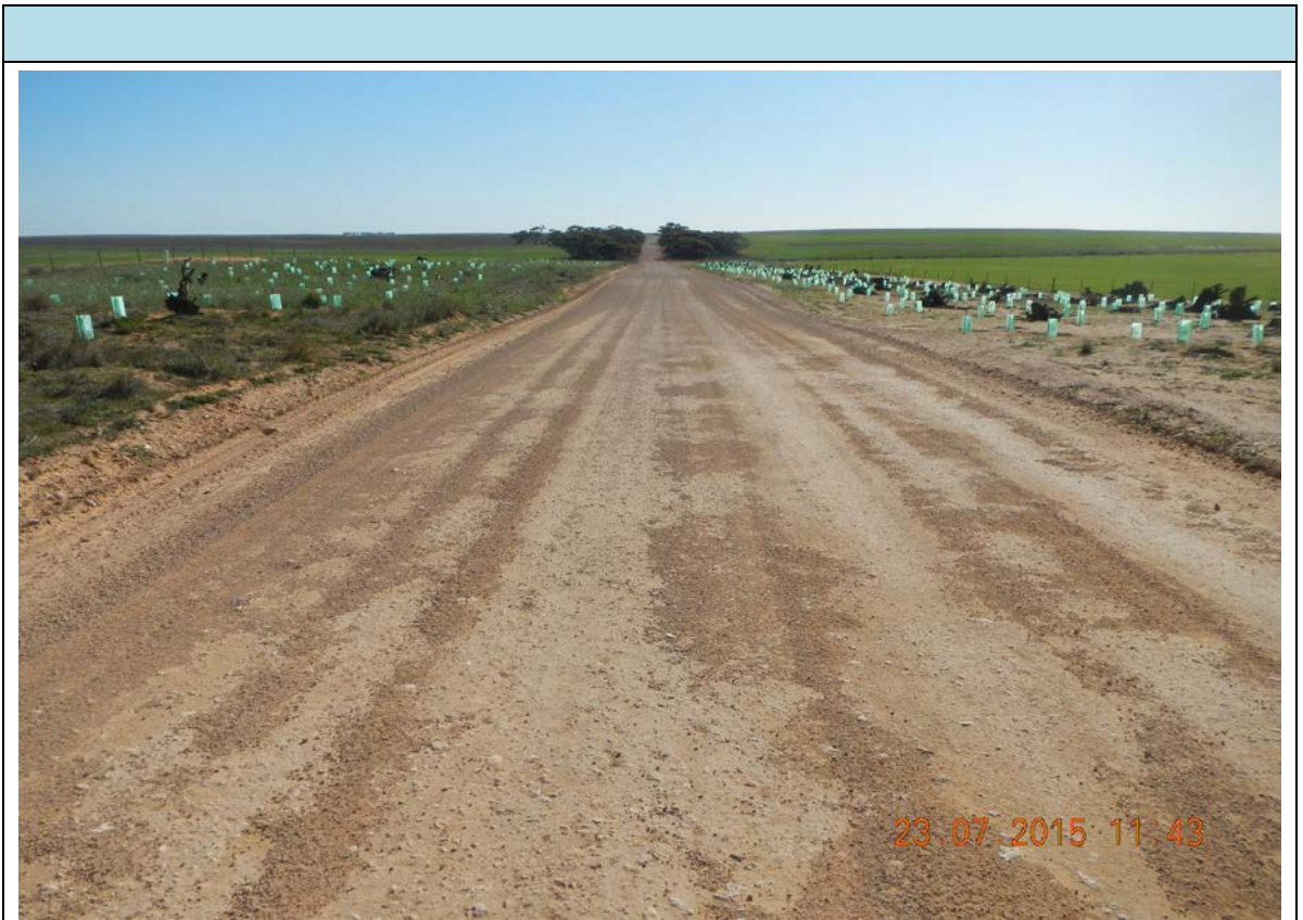
Photo 8: Reinstated gravel pavement and native vegetation along Knights Well Road
