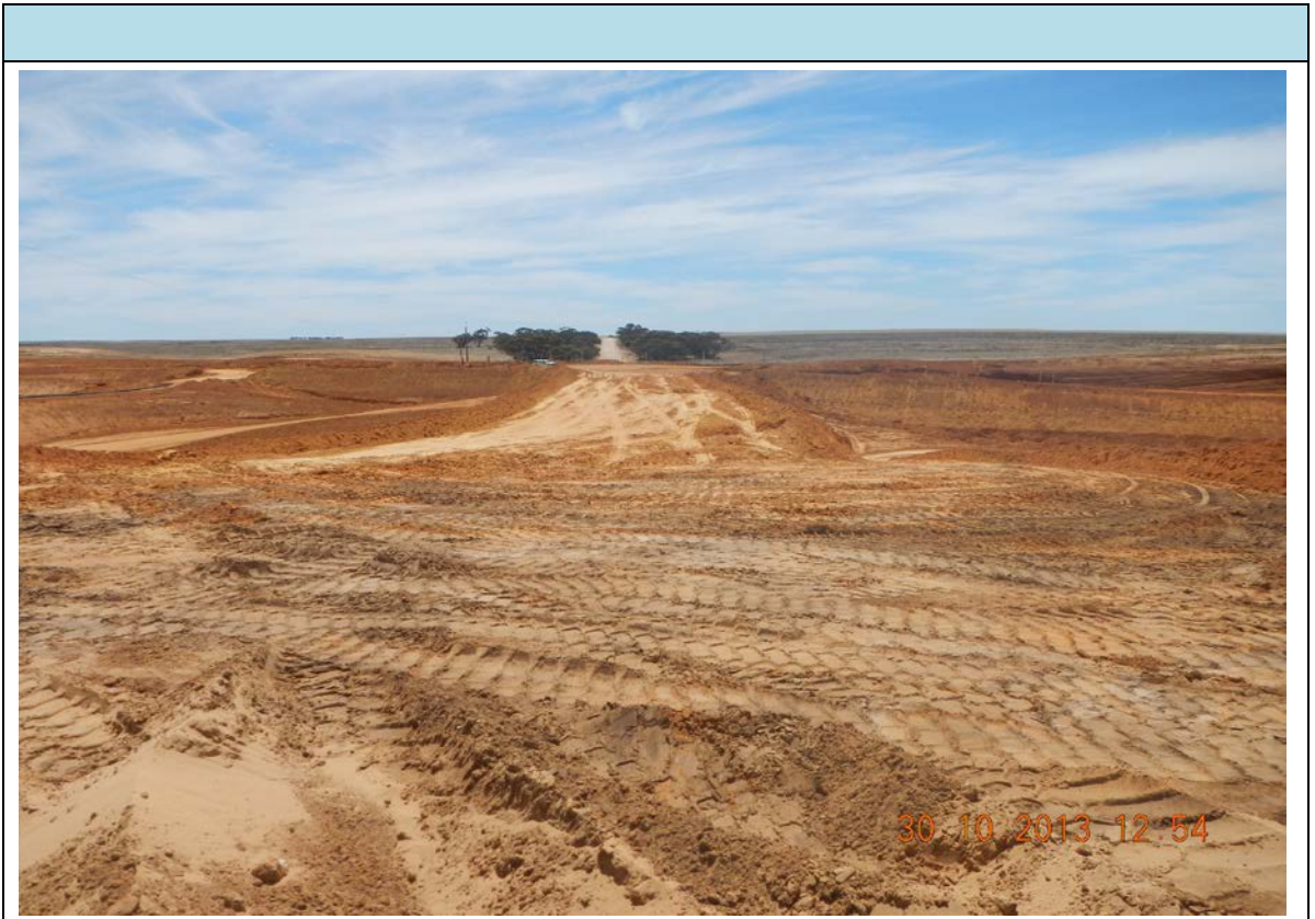
Photo 7: Mining through Knights Well Road
