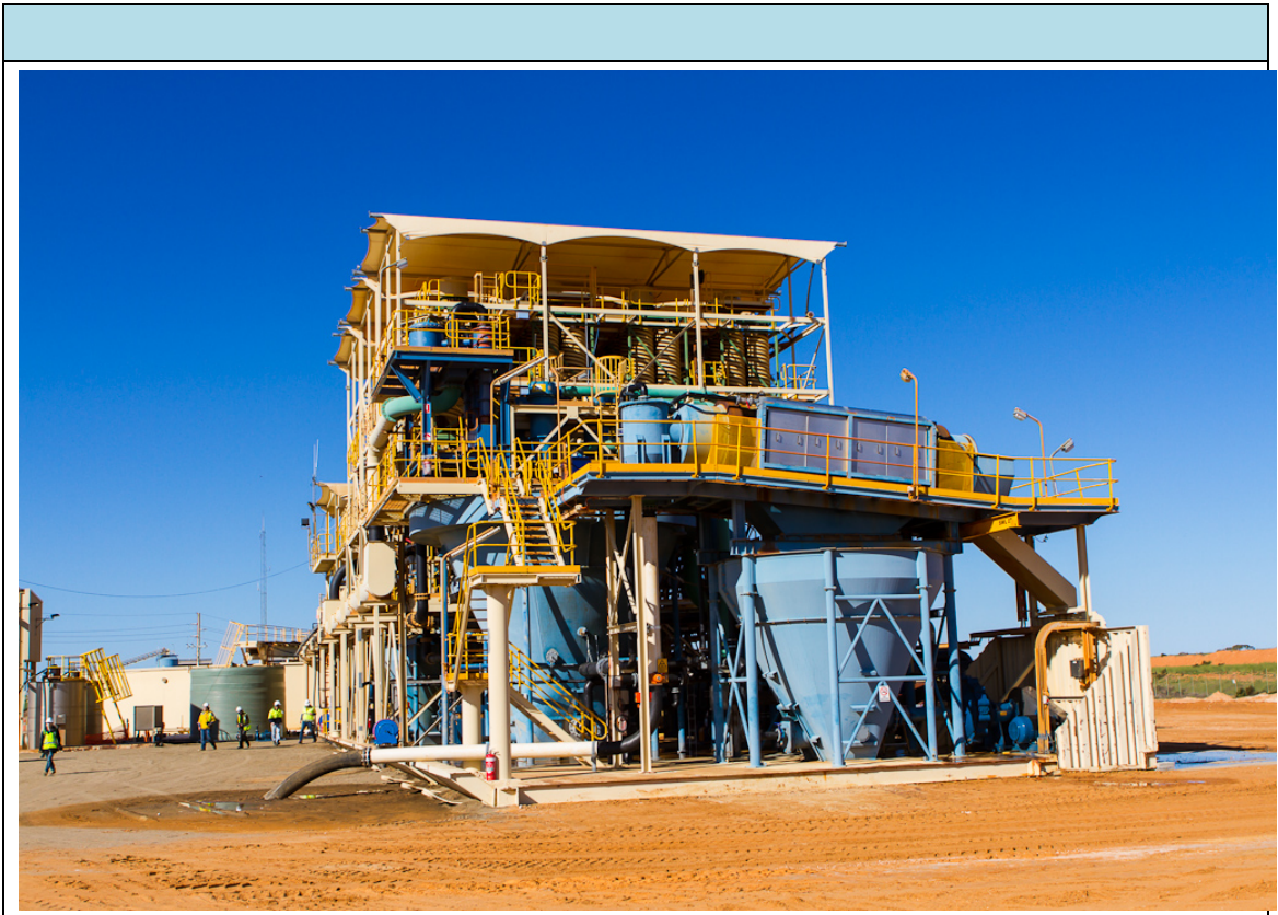
Photo 3: Mindarie project primary concentration plant
