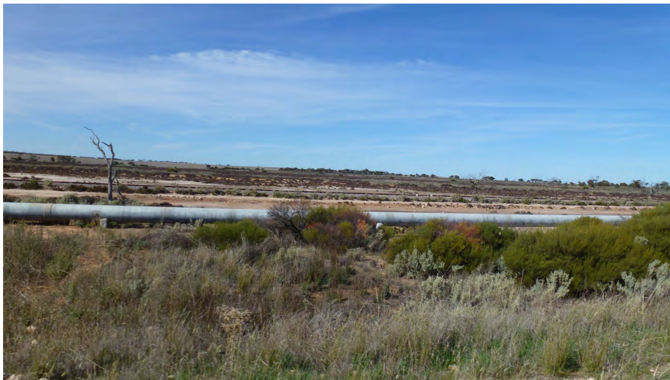
Photo 3: Swale next to Tod Highway, main pipeline and railway between Warramboos and Kyancutta Eastern side view
