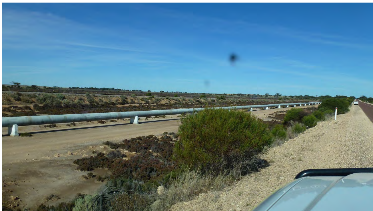
Photo 2: Swale next to Tod Highway, main pipeline and railway between Warrambo and Kyancutta Eastern side view
