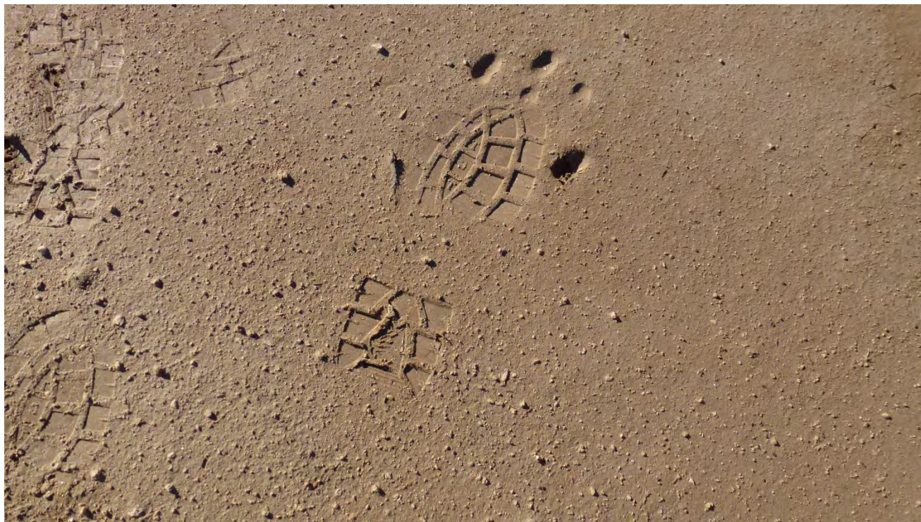
Photo 17: Detail of surface of the swale
