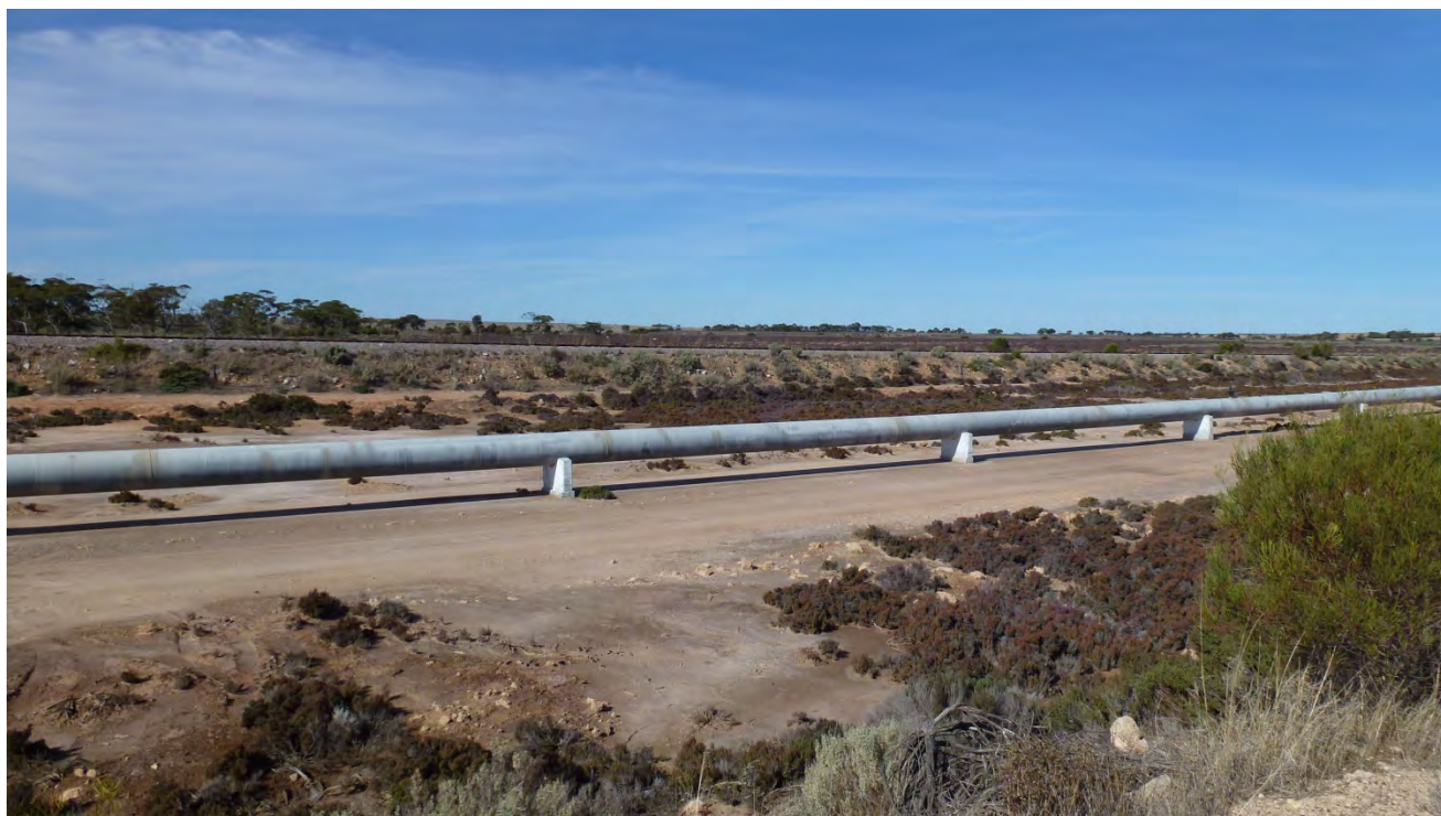
Photo 1: Swale next to Tod Highway, main pipeline and railway between Warrambo and Kyancutta Eastern side view
