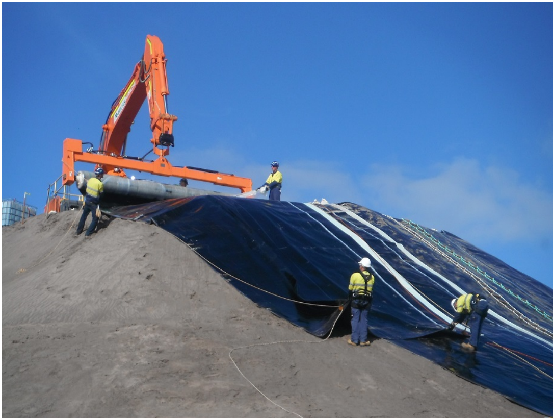
Plate 13 BGM installation
