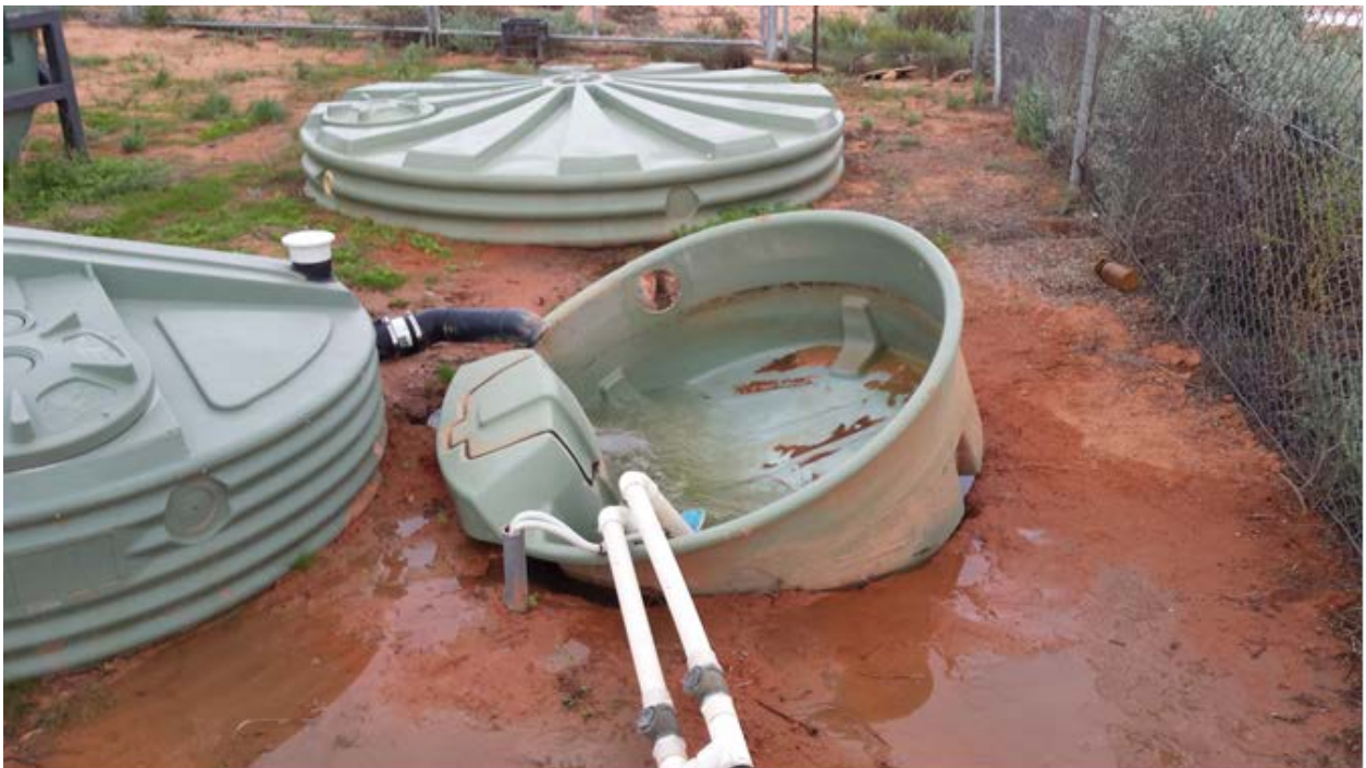
Plate 15 Overflow of wastewater from the humus tank at Jacinth village
