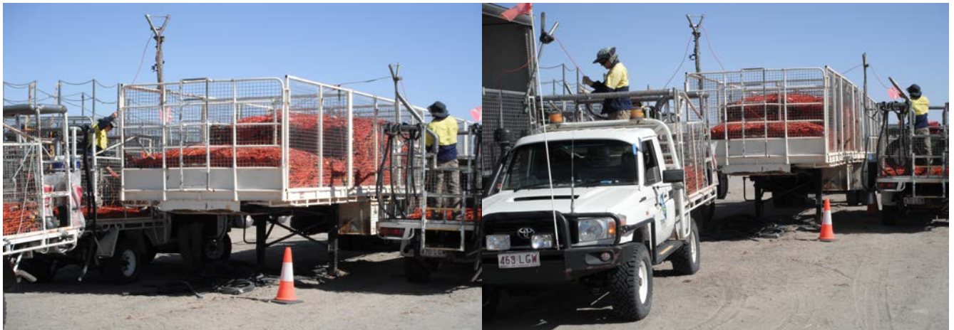
Pulling cable and phones off the spread truck at the start of the job
