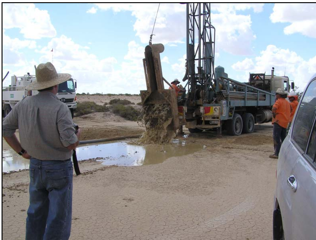
Picture # 6- 4: emptying the mudpit at the completion of a hole.
