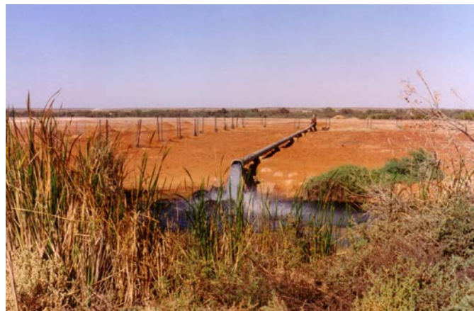
Clayton 2 Bore headworks (pillar at rear), outflow pipe and storage pool, Clayton Pastoral Station. This artesian water is initially hot (>75 °C) and is used for stock supply after cooling in the storage pool. Note the condensing steam near pipe outflow. The aquifers are Algebuckina Sandstone and Cadna-owie Formation. (Photo 410053)
