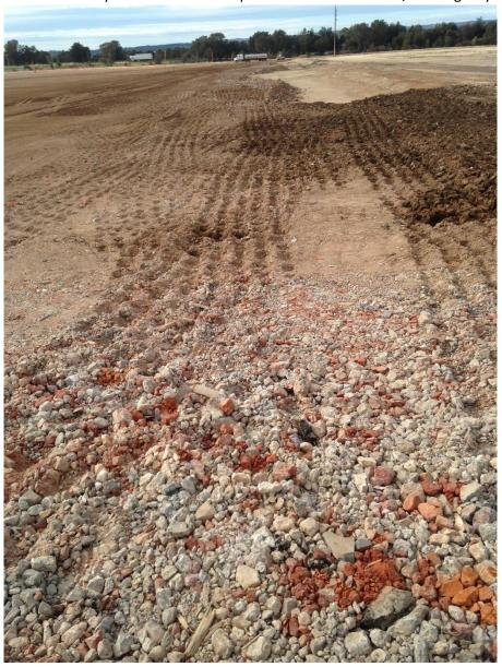
This photo taken on 4 July 2018 shows the 2000 m2 mound of imported fill placed on the base filter / drainage layer
