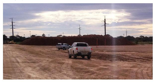
This photo taken on 4 July 2018 provides a view to the north east from the south west corner of the area on which the base filter / drainage layer had been placed and was in the process of being compacted by a small sheepsfoot roller – visible in the photo
