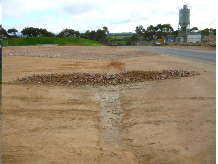
Plate 12: View of Silt traps at front entrance drive way, Western side
