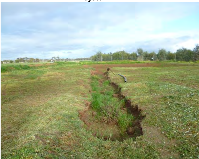
Plate 15: View of drain into Sediment Dam
