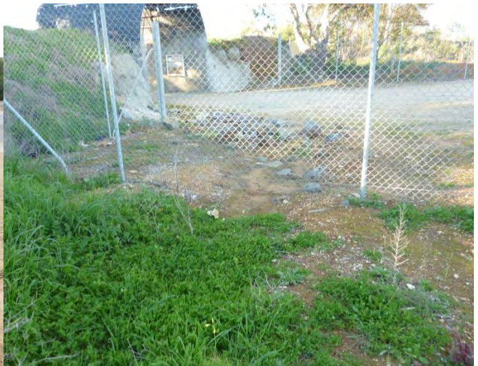
Plate 14: View of Surface drainage system into visitors viewing area
