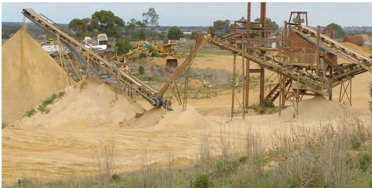
Figure 50: Pre-mining Site Showing Crushing and Screening Plant
