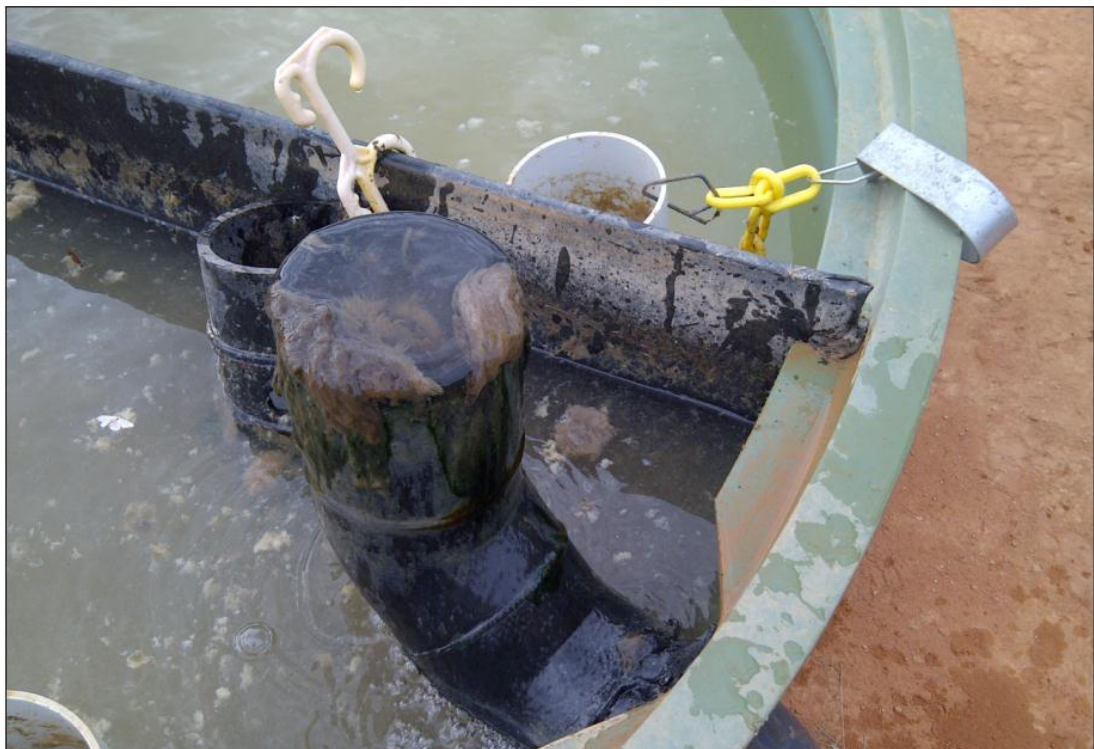
Figure 30 – Plunging and purge of humus draw-off pipe to reinstate normal flow
