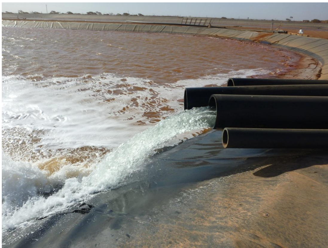
Figure 19 – Groundwater return to process water dam
