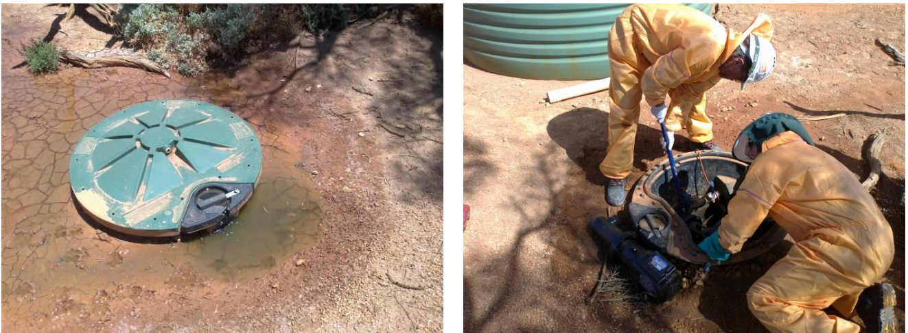
Figure 29 – Septic overflow from receiving tank and replacement of macerator pump
