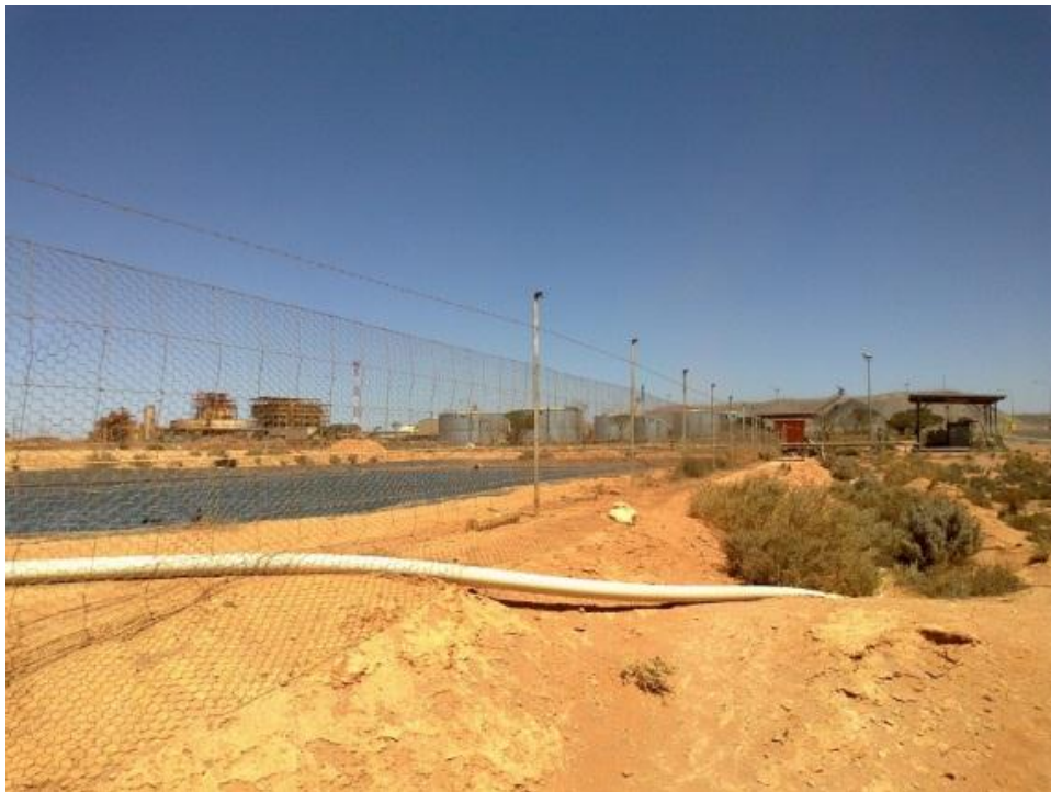
Figure 13 – Chicken wire upgrade to existing process water pond cyclone fencing
