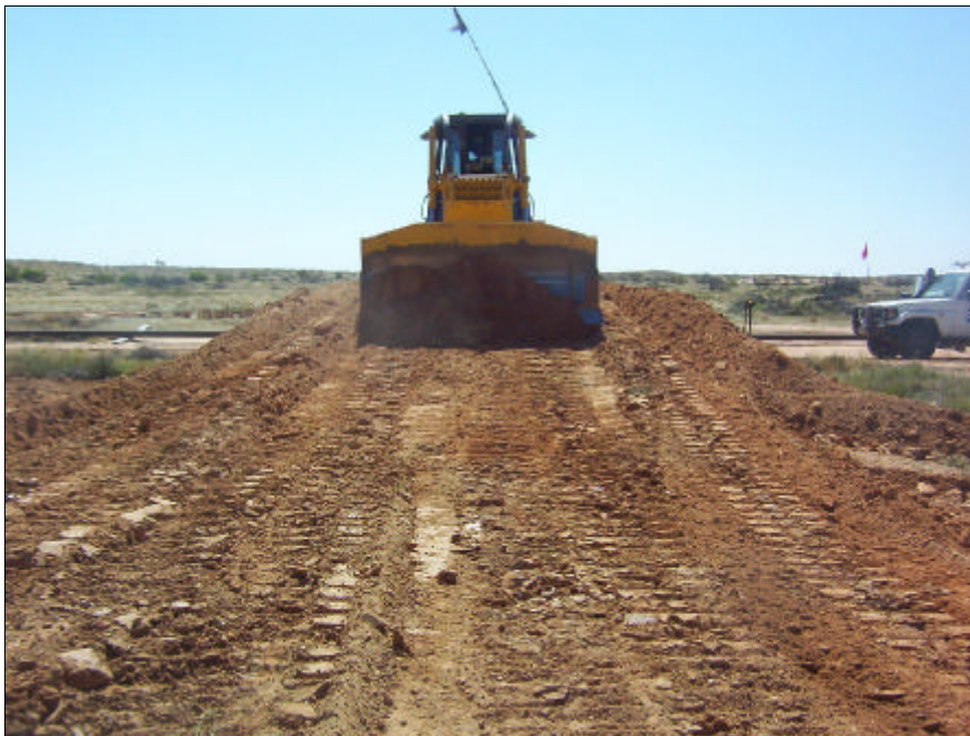
Picture # 6- 2: constructing one of two ramp over the Tantana oil pipeline.
