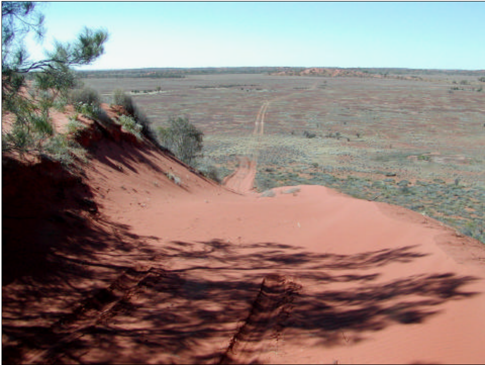
Picture # 3: Line BC03-14 looking north across a gibber plain; note the dangerously blown-in side-cut on the large dune in the foreground.
