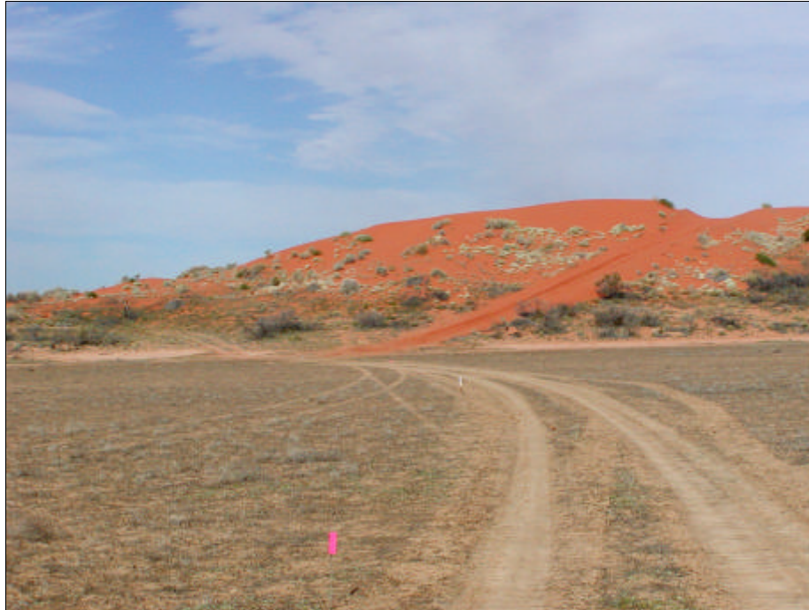
Picture #6- 4: large dune on line BC03-10 where the dozer operator made two mistakes; the first was choosing the highest part of the dune to cross and the next was a climbing turn.
