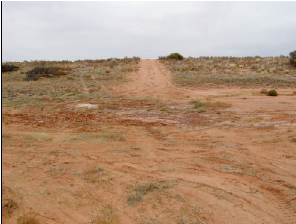
Picture # 5- 2: Example of an uphole site; cuttings are spread but mud is still evident.
