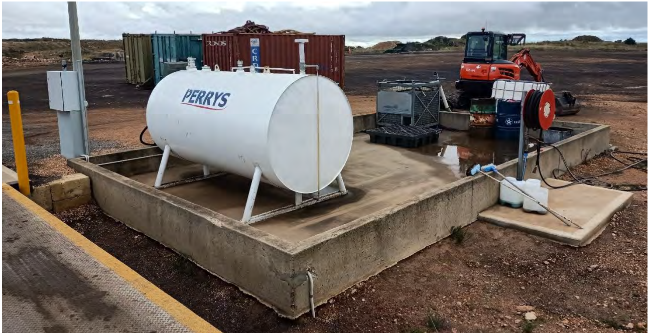
Plate 12 – The fuel and waste oil concrete banded storage area
