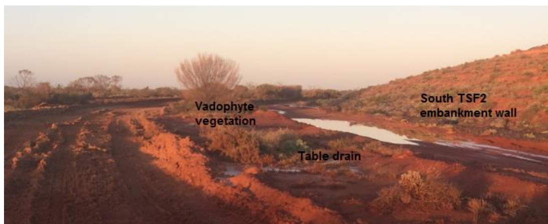
Plate 1 Wet ground near south embankment wall of TSF
