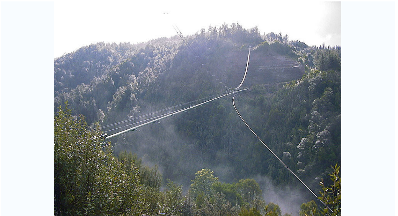
Figure 18: Savage River Mine slurry pipeline 366 m bridge span at 167 m above the Savage River (Source http://www.highestbridges.com/wiki/index.php?title=Savage_River_Pipeline_Bridge , viewed 27 December 2013)
