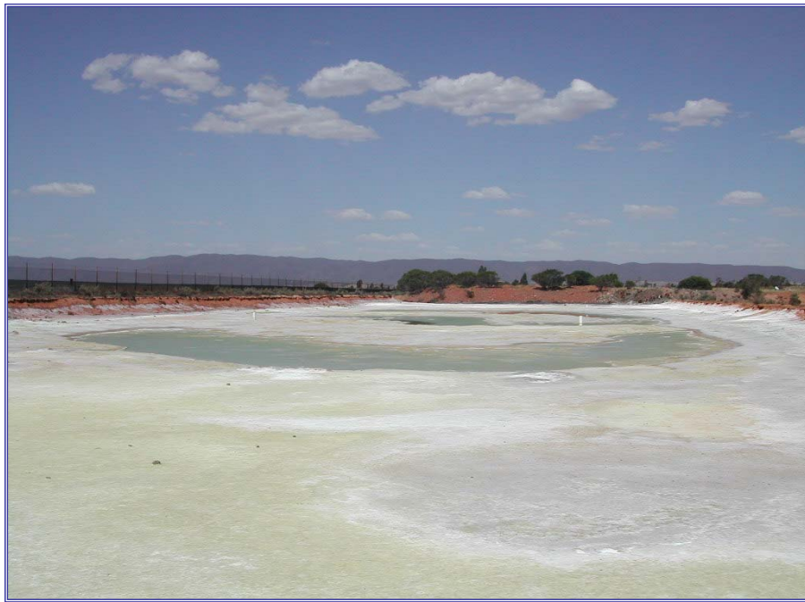
Figure 7 Easterly view of uncovered portion of dam 6
