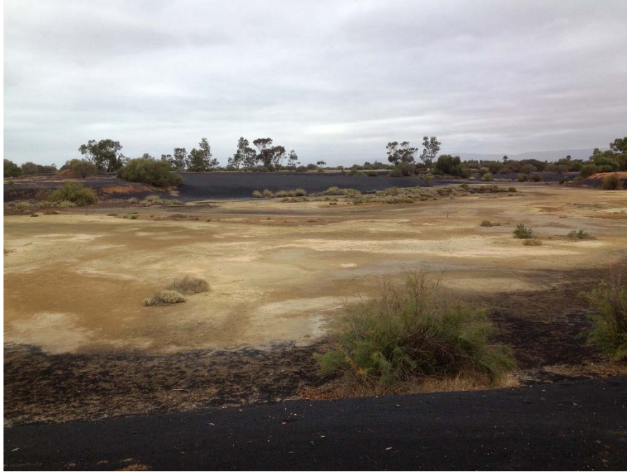
Figure 6 Tailing Dam 1 covered in Smelter Slag in background with evaporation pond in foreground
