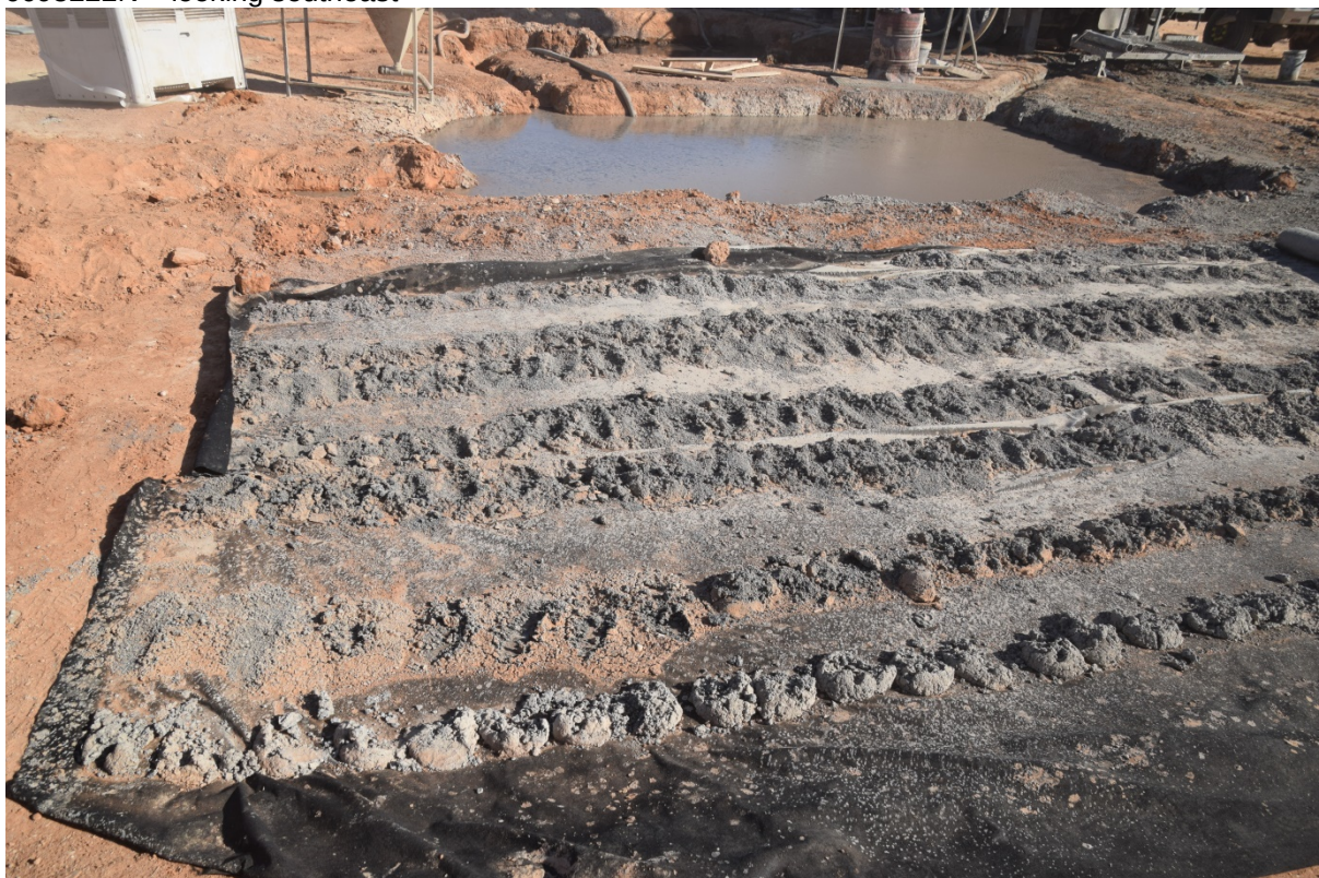
[Plate 4] WO-17-01 Drill Site – Pre-collar samples laid out on plastic sheet. Drill cuttings were placed in sump after collection of representative samples.
