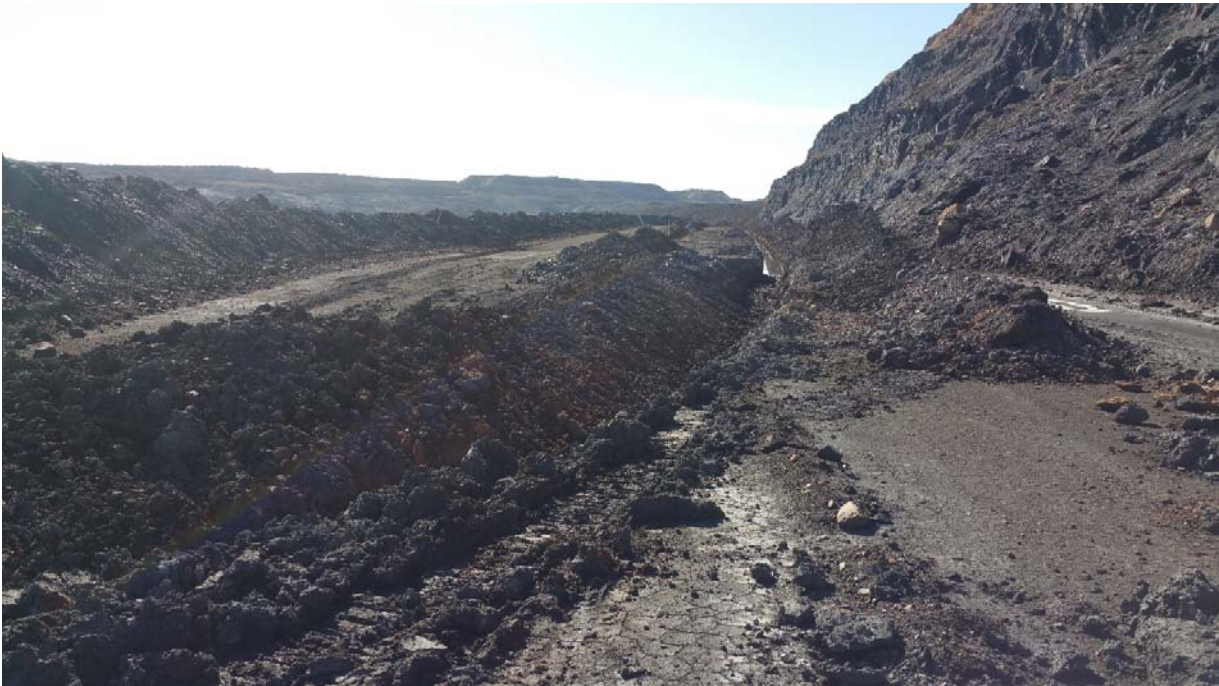
Figure 1.5 Excavated drain on Main Series EL140 haul road
