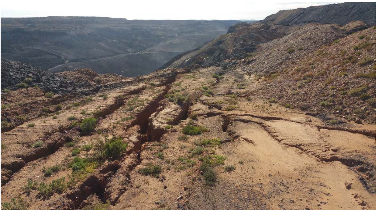
Figure 1.6 Previously known cracking of M14 high wall
