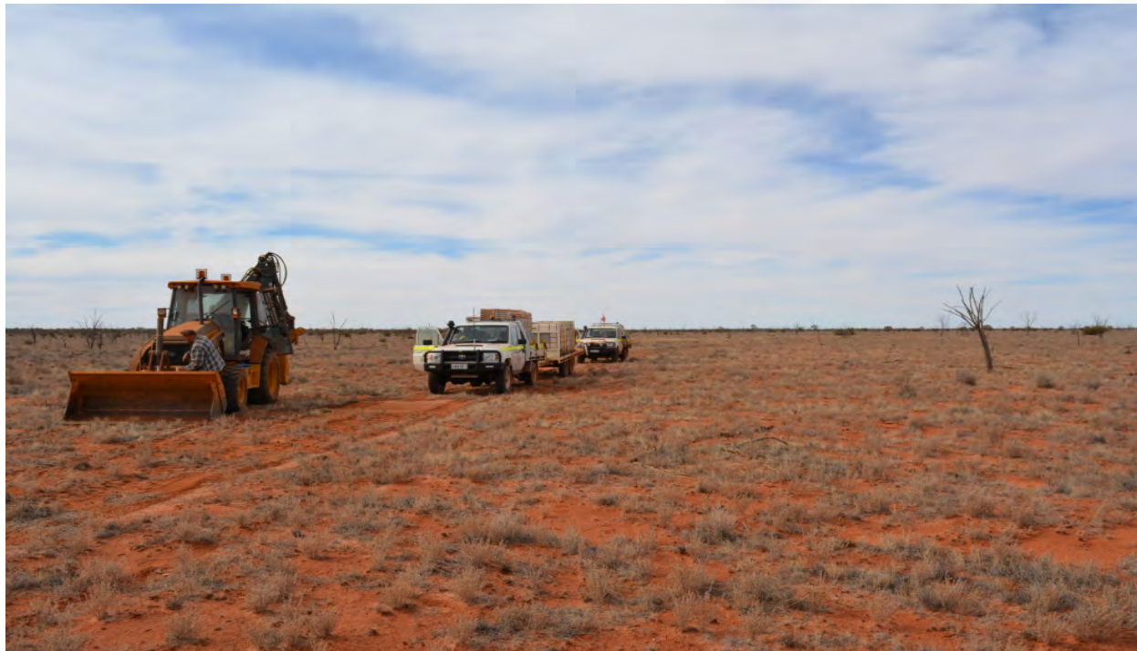
Photo 1: Backhoe used for clearing track and consumables being transported to site.
