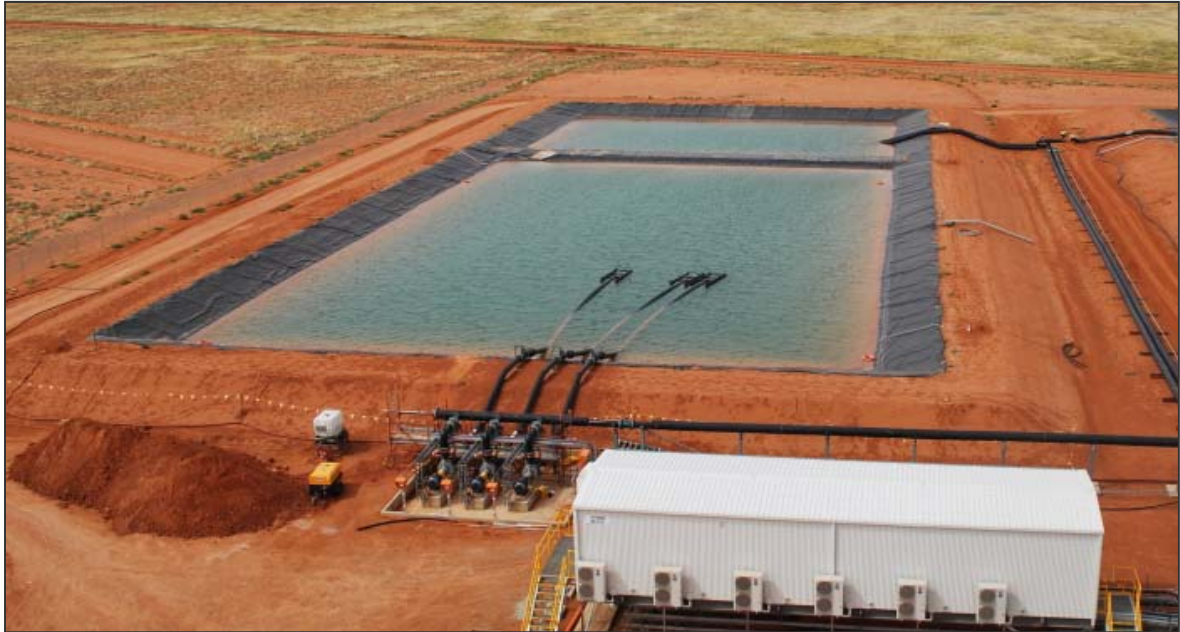
Plate 4.4 Barren leach solution pond at Honeymoon mine
