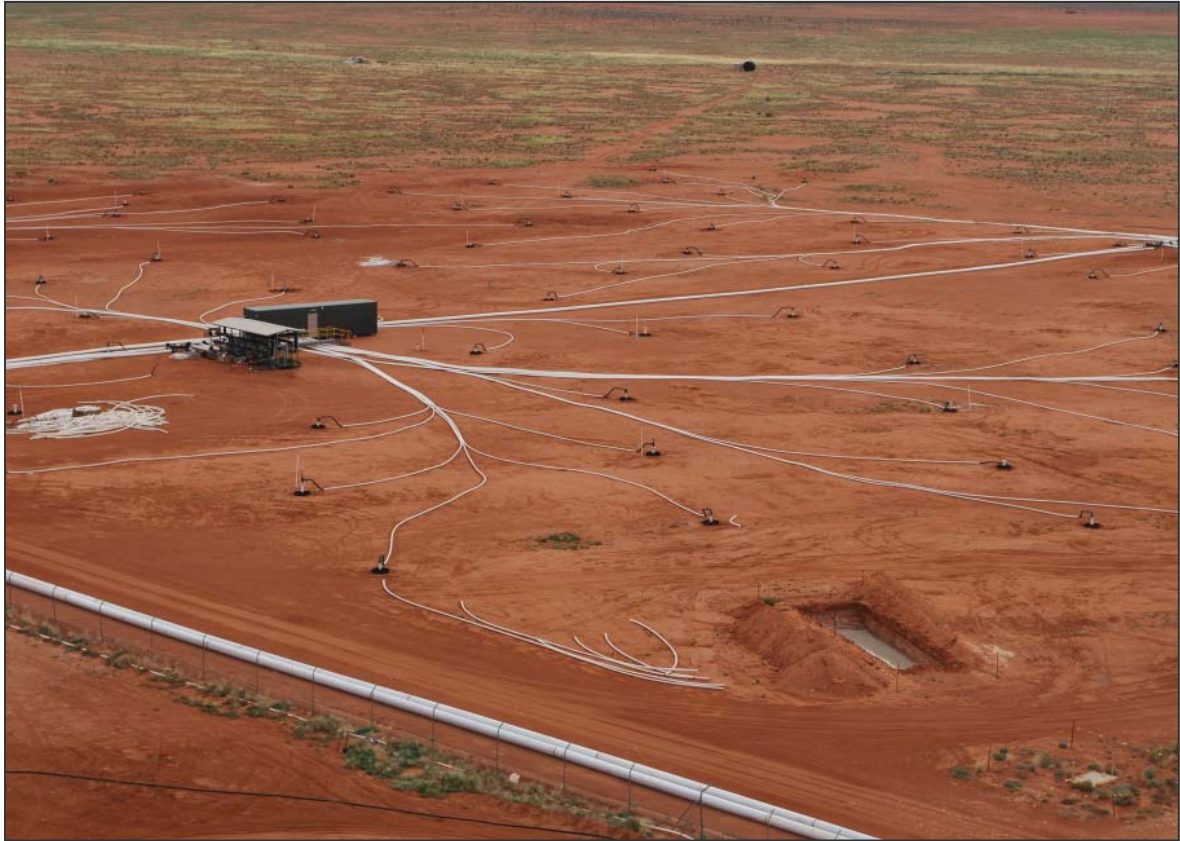
Plate 4.1 View of Wellfield C
