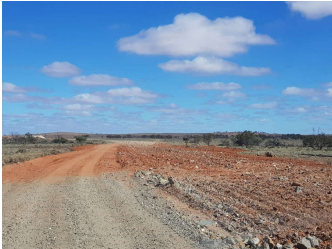
Figure 14: Vertigo Haul Road rehabilitated for light vehicle access only
