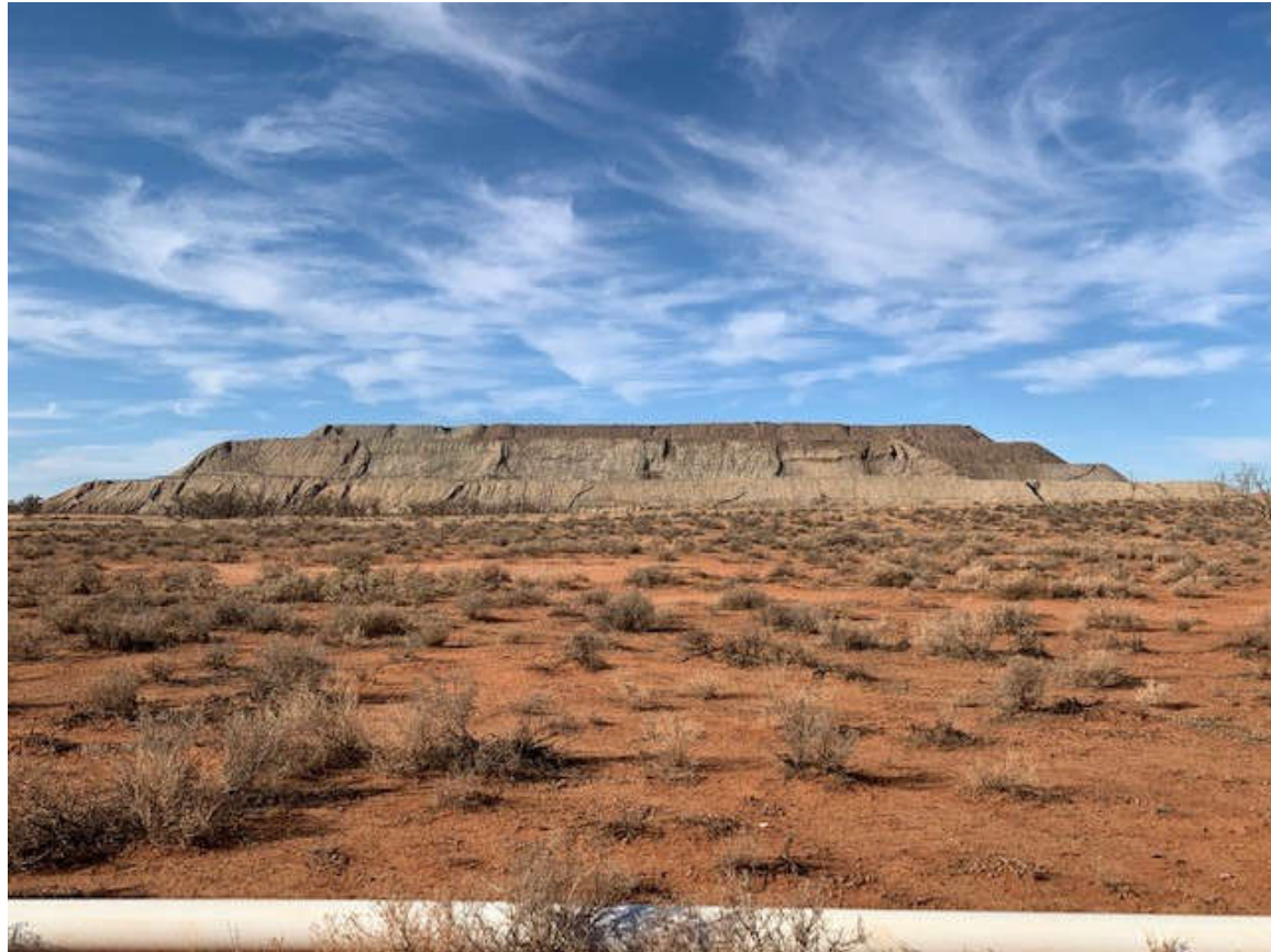
Figure 5: Photo of completed Heap Leach looking south - three lifts (end-2019)
