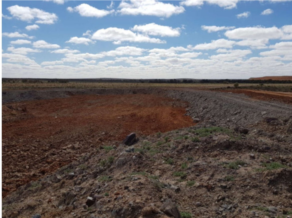
Figure 17: Vertigo pit apron inside abandonment bund: topsoil spread, ripped and seeded.
