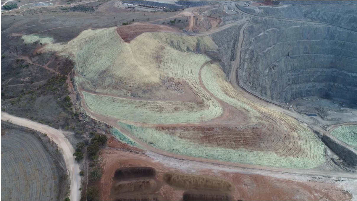
Figure 3-30 - Backfilled Nugent pit during hydroseeding (light green areas) May 2018
