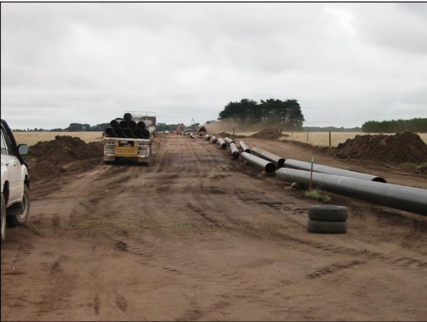
Plate 3-7: Pipeline delivery (left) and stringing (right)
