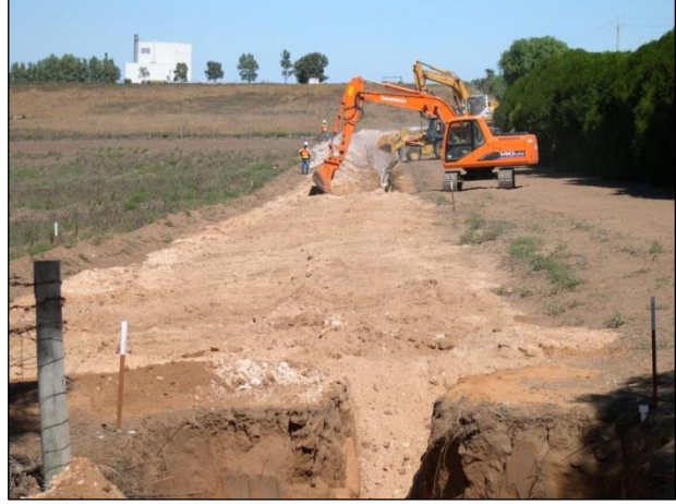
Plate 3-10: Padding (left) and backfill (right). (Left: large diameter pipeline construction. Right: small lateral construction)
