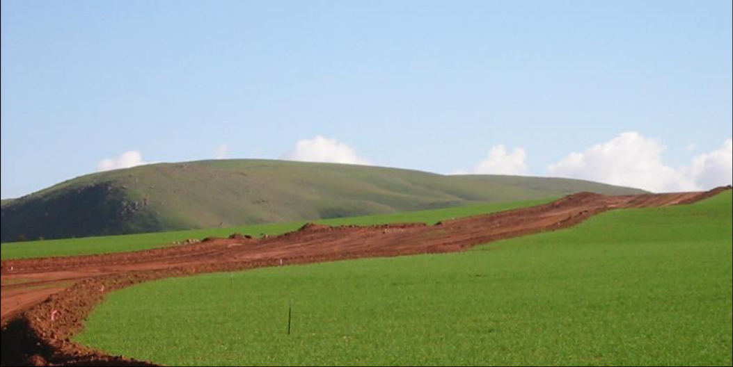
Plate 3-6: Clear and grade (large diameter pipeline)
