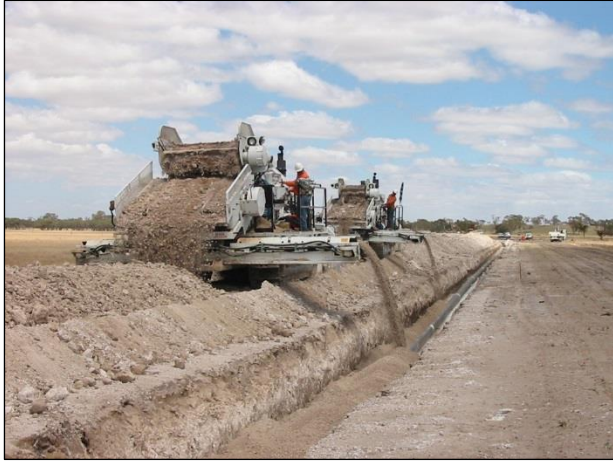
Plate 3-10: Padding (left) and backfill (right). (Left: large diameter pipeline construction. Right: small lateral construction)
