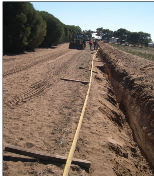
Plate 3-9: Lowering in (Left: large diameter pipeline construction. Right: small lateral construction)
