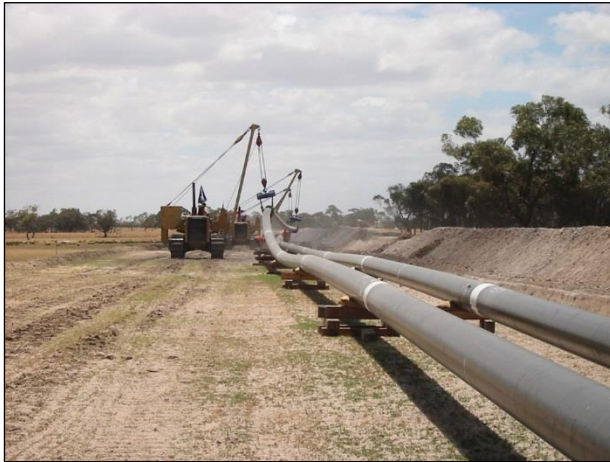
Plate 3-9: Lowering in (Left: large diameter pipeline construction. Right: small lateral construction)
