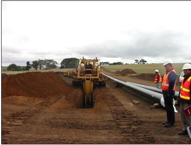
Plate 3-8: Trenching (Left: large diameter pipeline construction. Right: small lateral construction)
