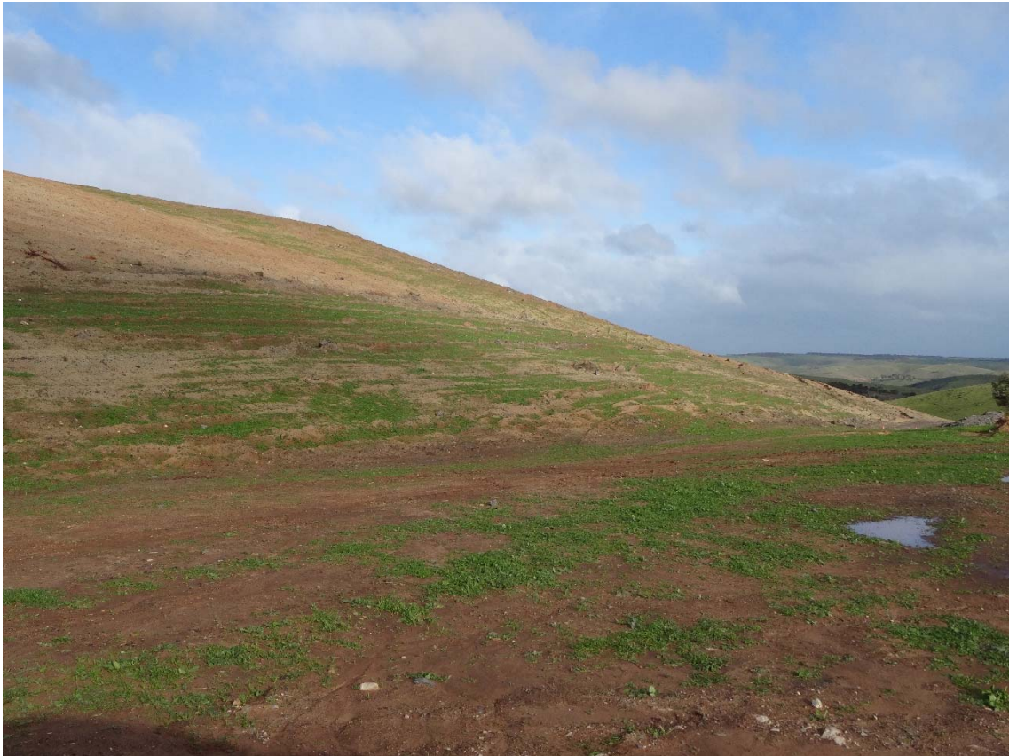
Figure 11 Reshaped IWL, with revegetated store and release cover comprising NAF waste rock and topsoil
