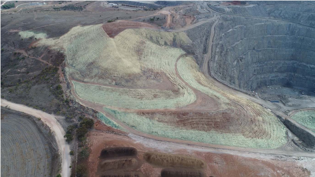
Figure 3-4 - Backfilled Nugent pit during hydroseeding (light green areas) – May 2018
