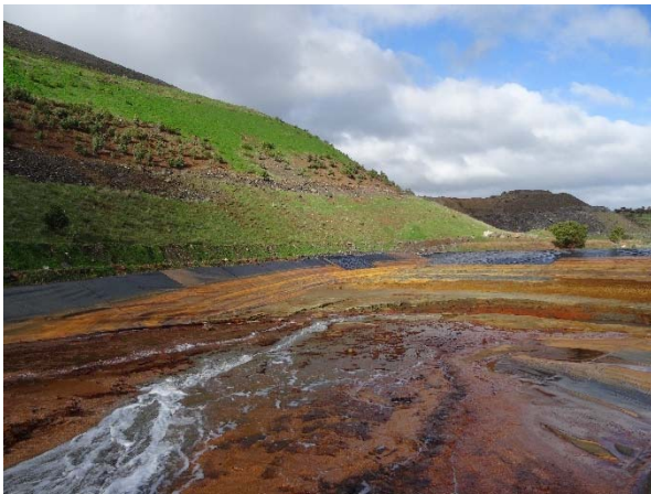
Figure 14 Variably textured and revegetated store and release cover on steep IWL slope below TSF and above RWD
