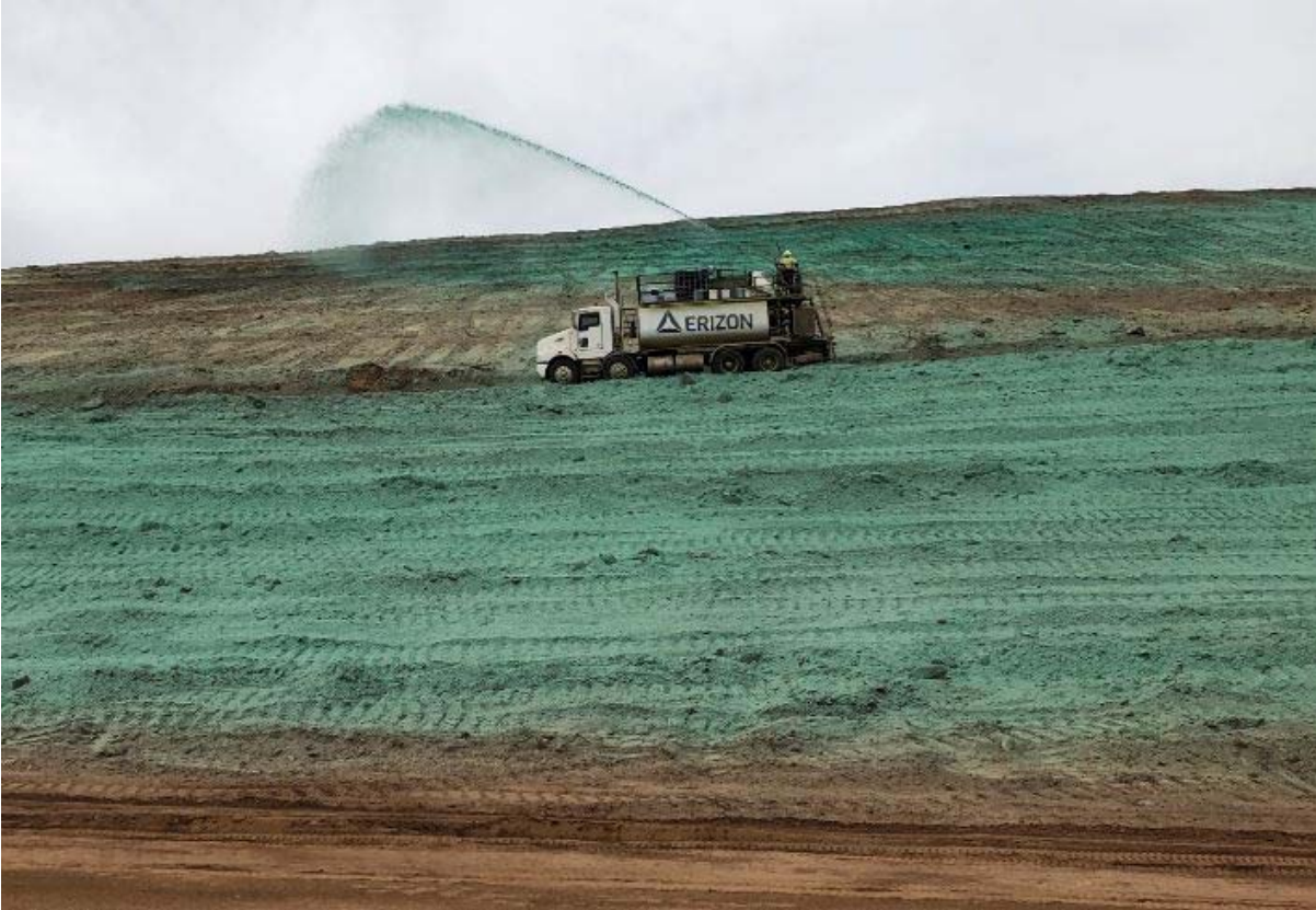
Figure 3-7 - Hydroseeding operations on the KCM IWL (March 2019)
