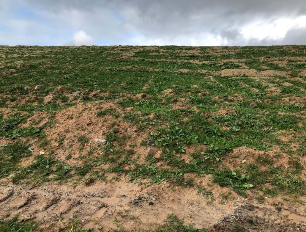
Figure 3-8 – Resultant vegetation germination 4 months after hydroseeding (August 2019)
