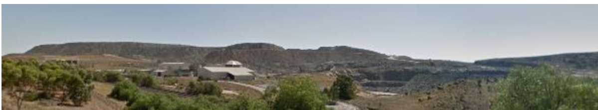
Plate 10: View from the trainline adjacent to the mine substation looking north west. Google (2019).
