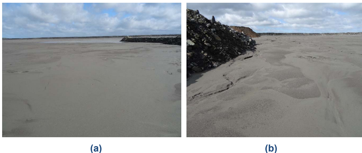
Figure 9 TSF, showing: (a) distant central decant, and (b) desiccated sandy tailings beach midway along access to central decant
