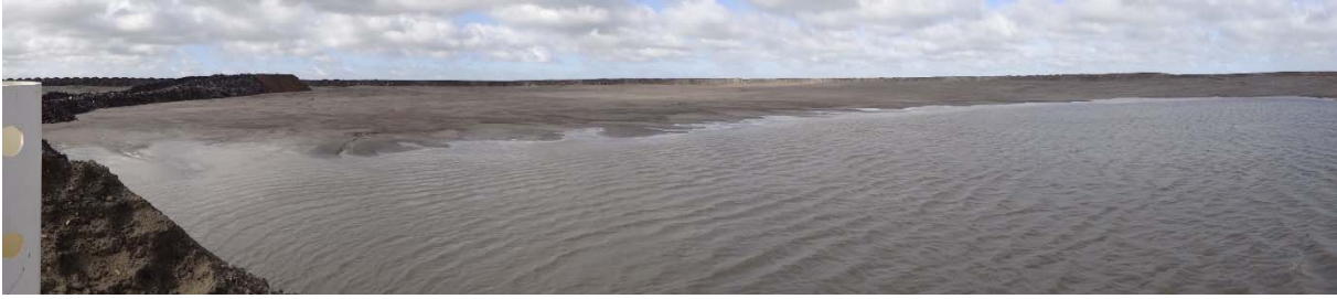
Figure 6 TSF from central decant pond
