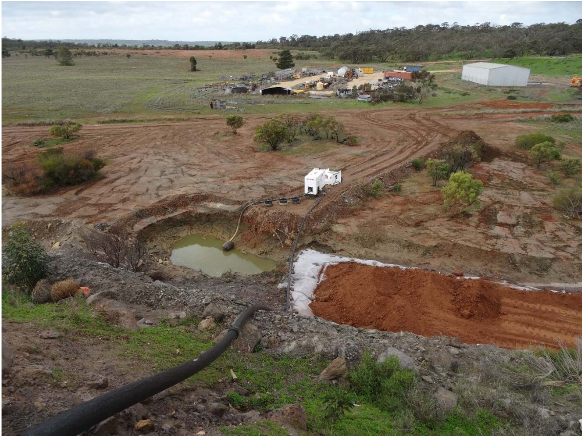
Figure 16 Surface expression of Groundwater at toe of IWL across surface of OTD tailings beach, which is being intercepted and drained
