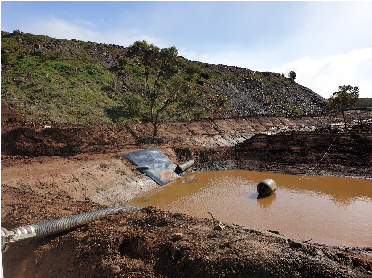
Figure 4 – Cut Off Channel and Seepage Interception Dam
