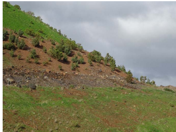
Figure 14 Variably textured and revegetated store and release cover on steep IWL slope below TSF and above RWD
