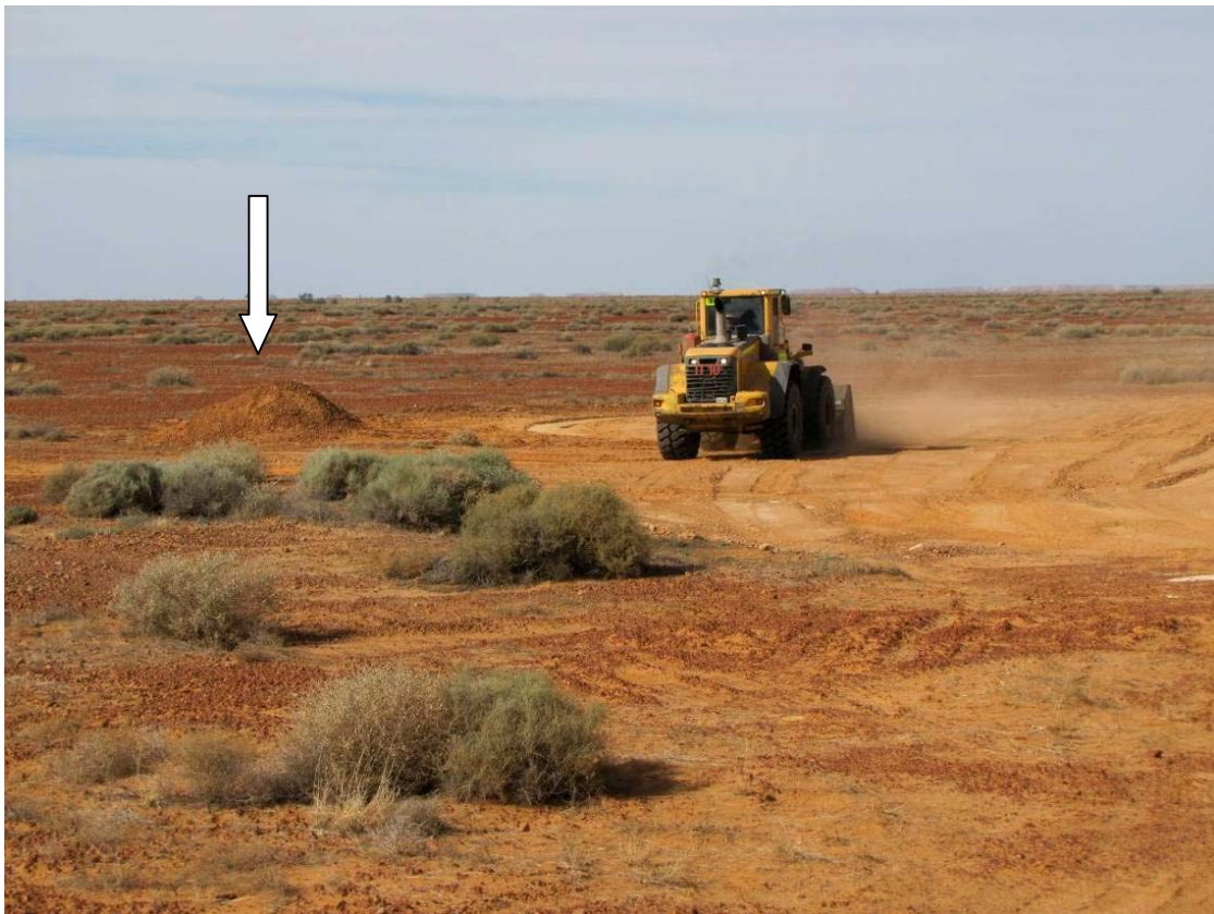
Photo 24: Levelling drill pad for CS001 prior to spreading topsoil. Topsoil heap arrowed.
