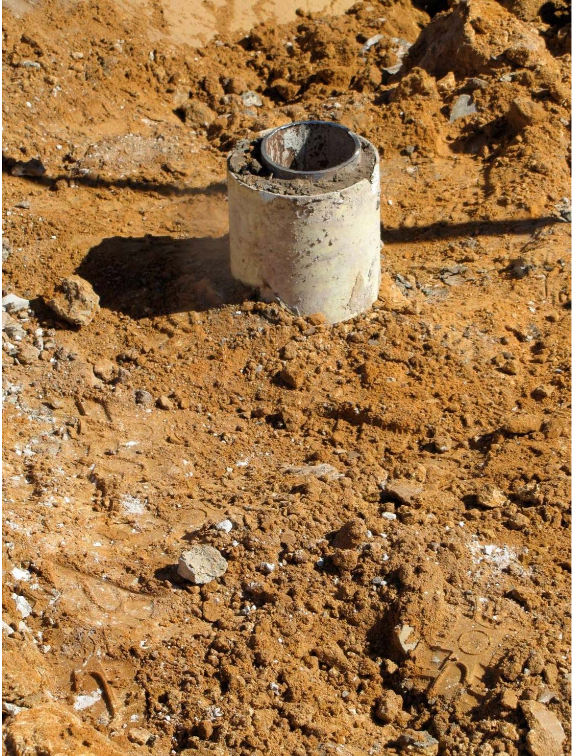
Photo 30: Casing for drillhole CS002 cut prior to burial below ground level
