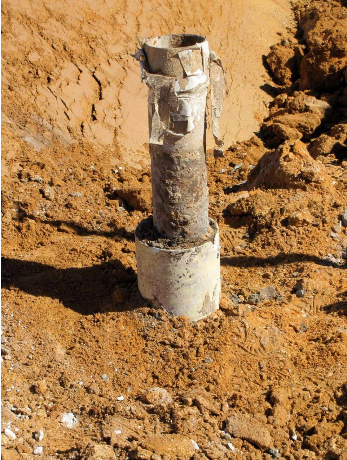
Photo 29: Casing for drillhole CS002 exposed for cutting below ground level.
