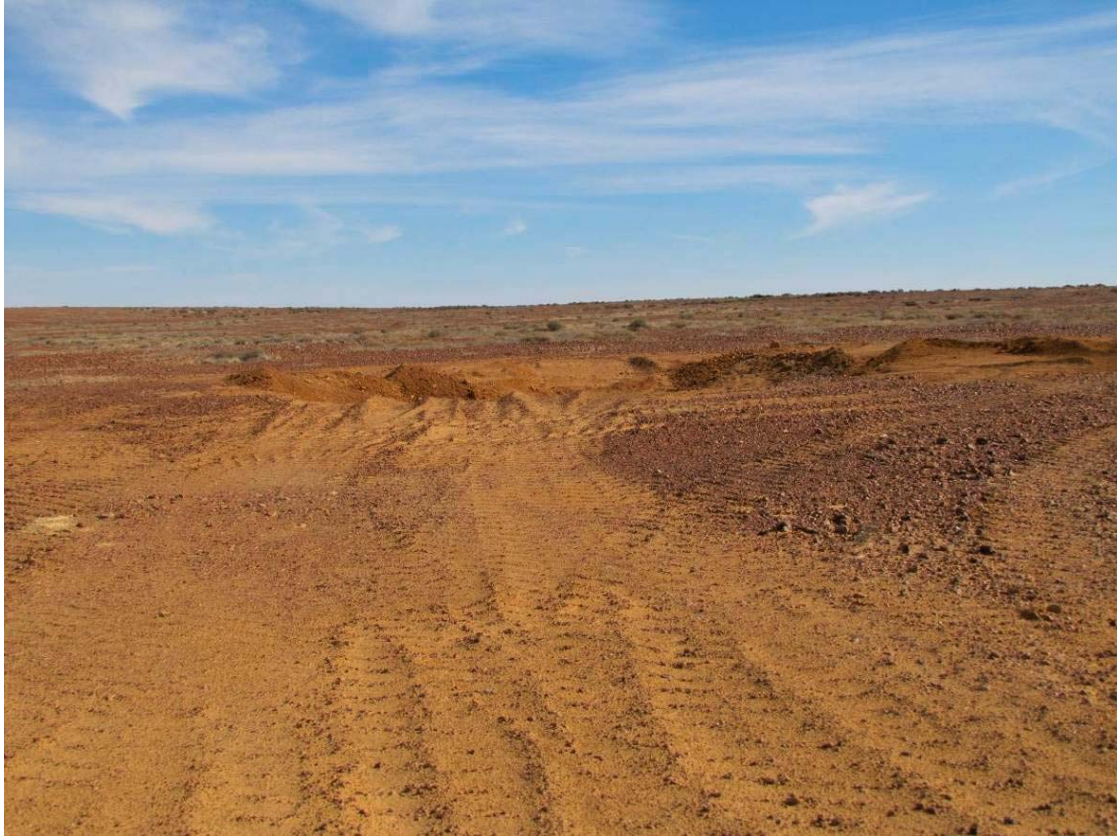
Photo 10: Borrow pit at 671586gdaE, 6732303gdaN before rehabilitation
