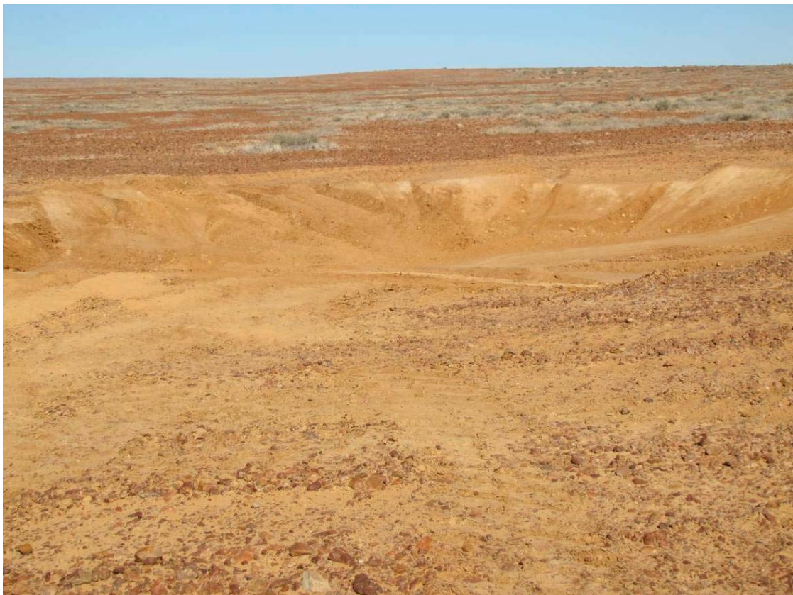
Photo 11: Borrow pit after rehabilitation showing "landscaping" with low gradient sides
