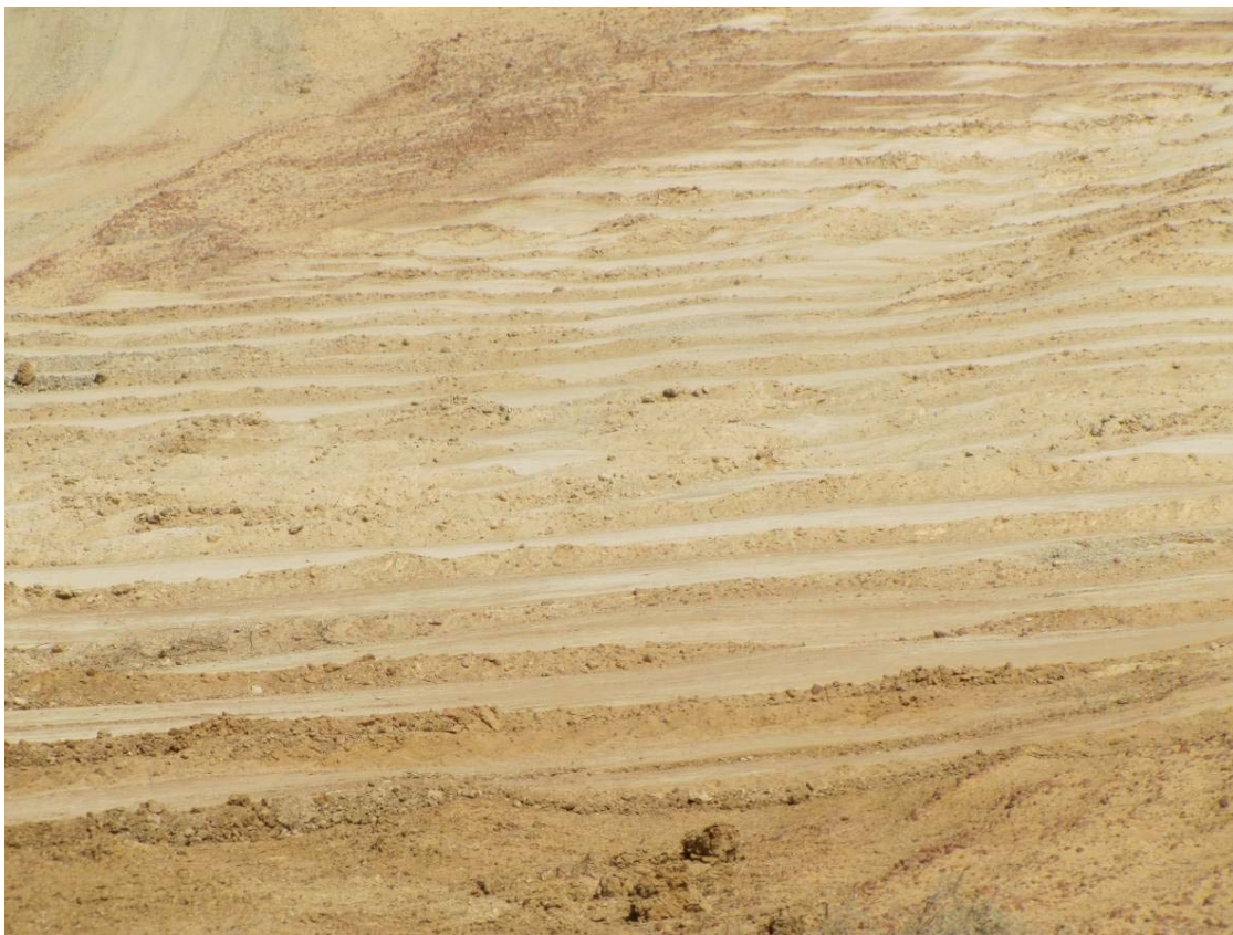
Photo 9: Closeup after rehabilitation showing mini bunding to prevent erosion
