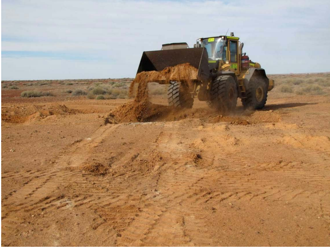
Photo 23: Backfilling sumps at drillhole CS001
