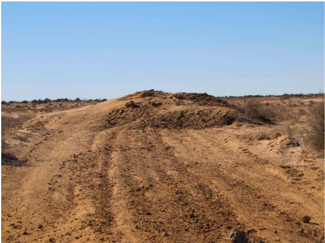
Photo 17: Access to drill pad CS 002 blocked by sand and gravel near entrance from station track
