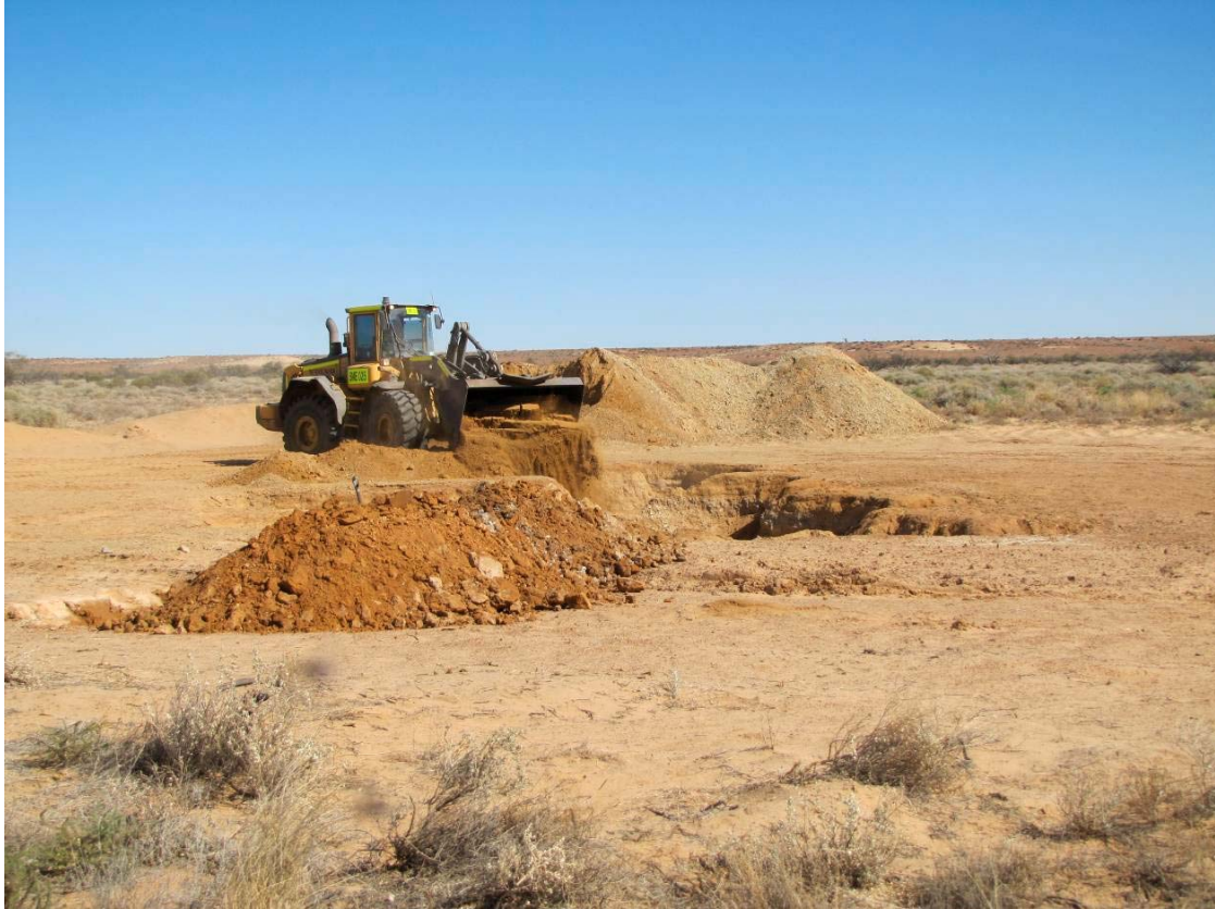
Photo 31: Backfilling sumps at drill pad CS002
