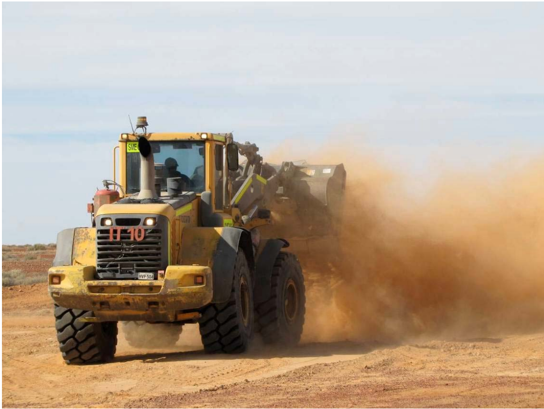
Photo 25: Spreading topsoil at drill pad CS001
