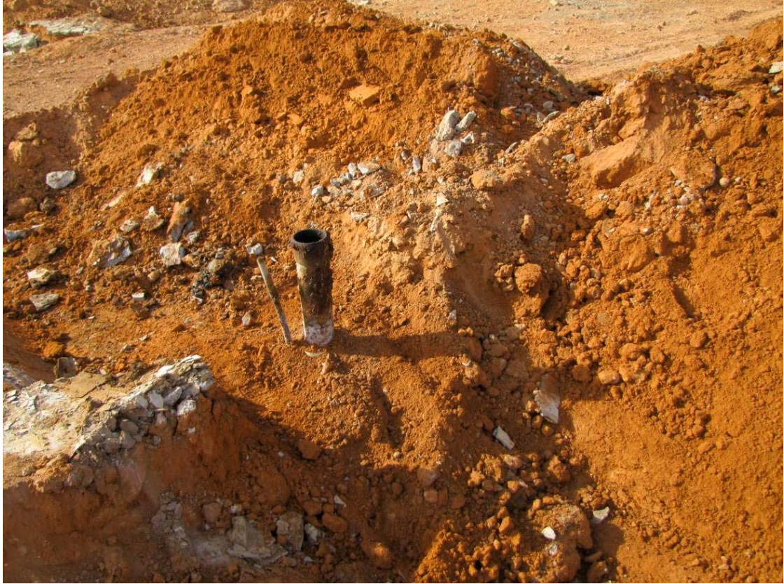
Photo 21: Drill collar for CS001 exposed prior to cutting below ground level.
