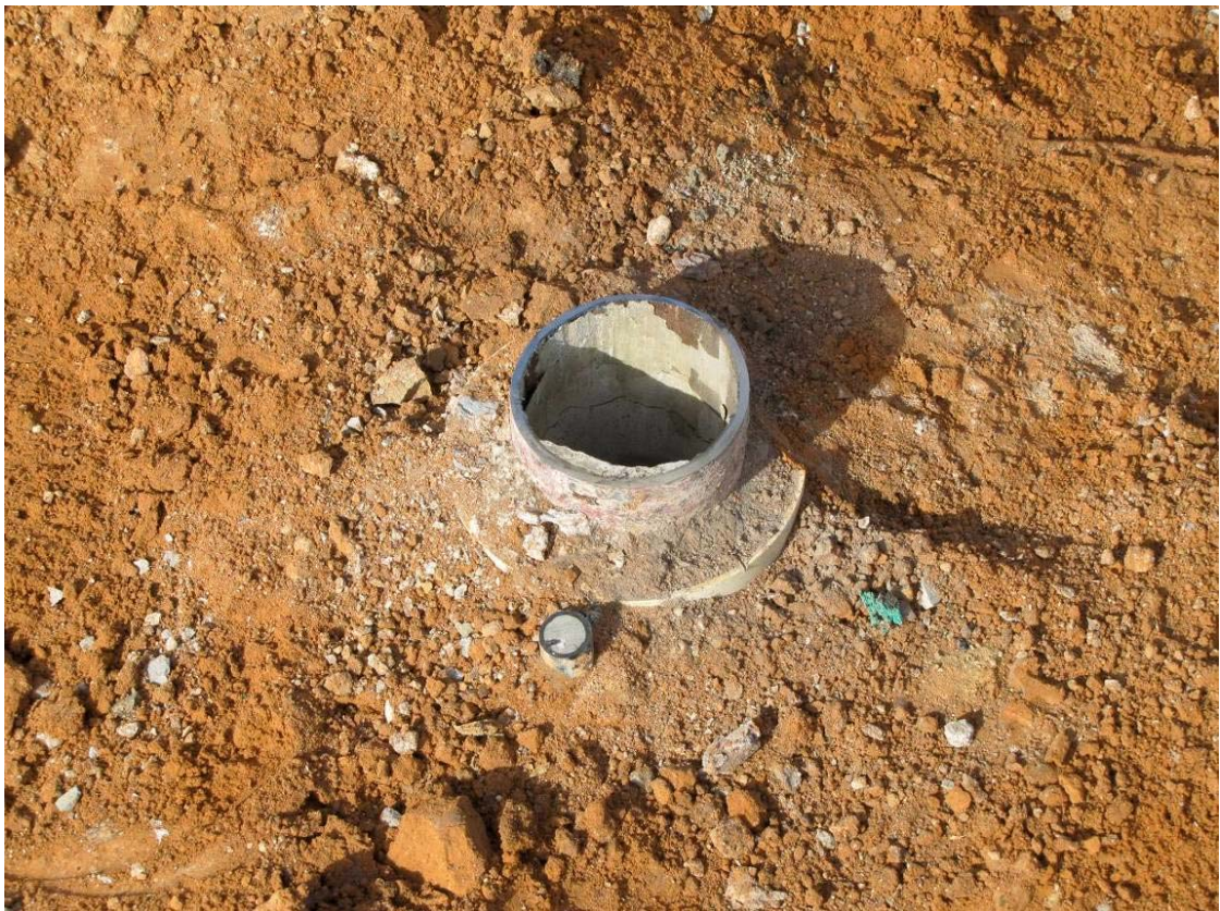
Photo 22: Drill collar for CS001 cut prior to burial below ground level
