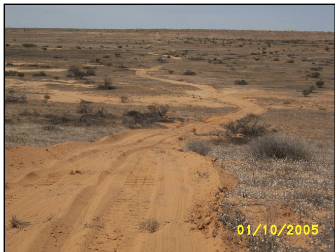
Example of Line Weaving by Dozers
