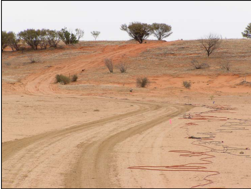
Picture # 3: line BC05-51 PEL 95; no bladework in swale, minimal cut on dune, weaving
