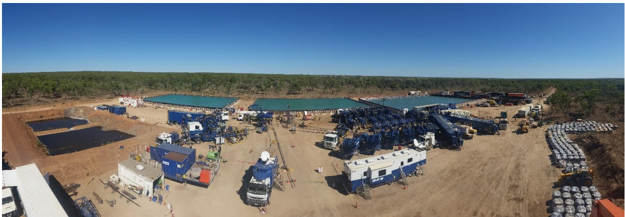
Plate 8: Fracture Stimulation Operations at Origin Energy's Amungee NW – 1H (Beetaloo Basin – Northern Territory). Note the temporary ponds in the background for stimulation activities. The ponds on the left were used for drilling purposes.
