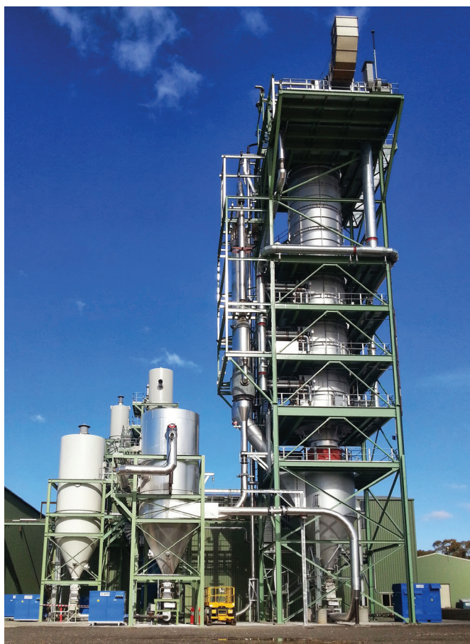
Figure 10 Calix Flash Calciner – commercial-scale demonstrator plant at Bacchus Marsh in 2013, and diagram of key components of the kiln system. (Courtesy of Calix; photo 417751).
