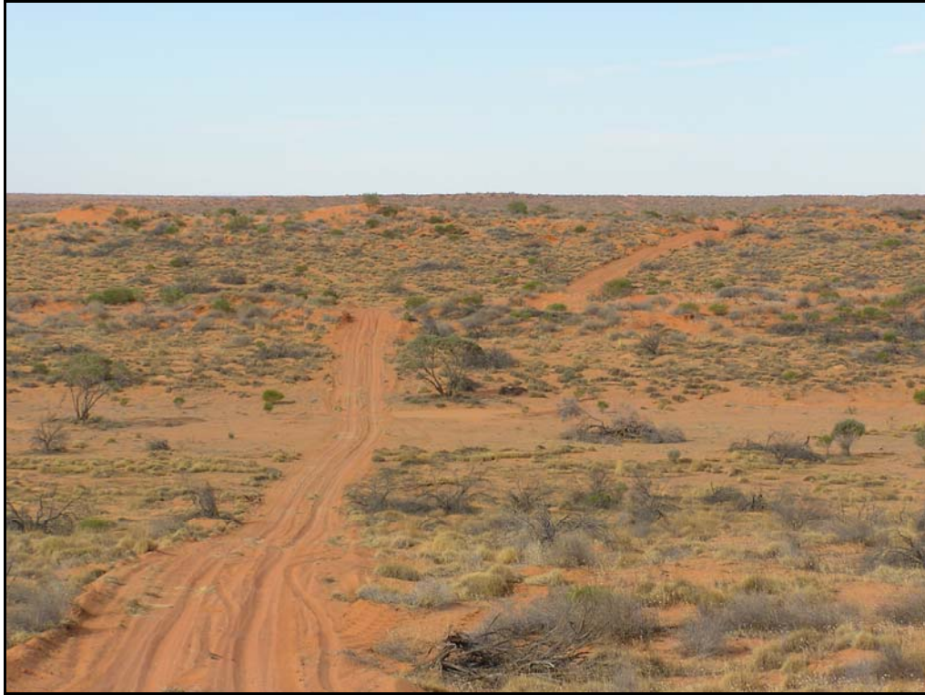
Picture # 7: line BC05-13; offset dune cuts break line of sight
