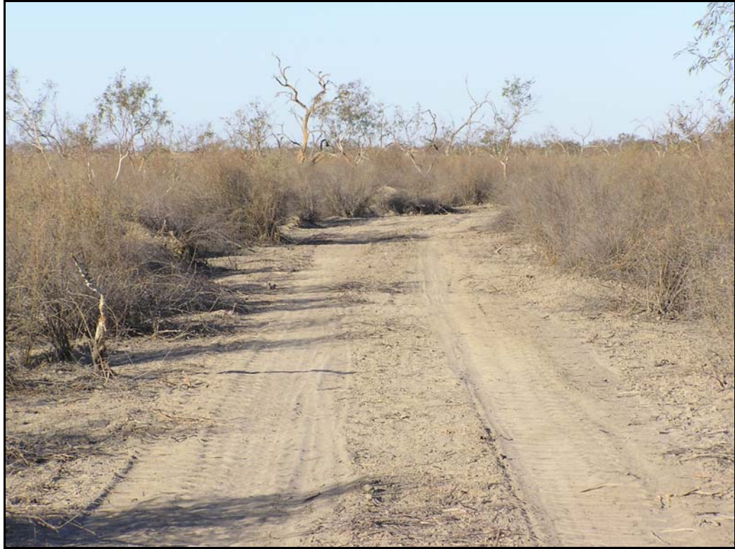
Picture # 13: line passes through a patch of lignum and swamp canegrass on line BC05-38; no windrows and rootstock left in place
