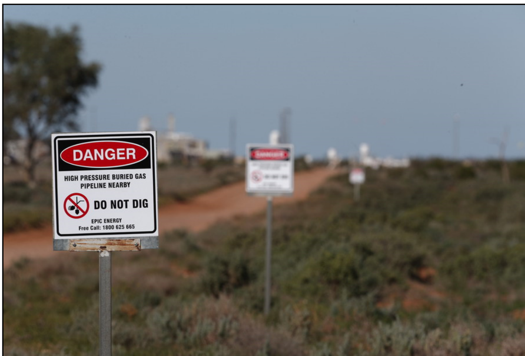
Plate 1: Pipeline Marker Signs
