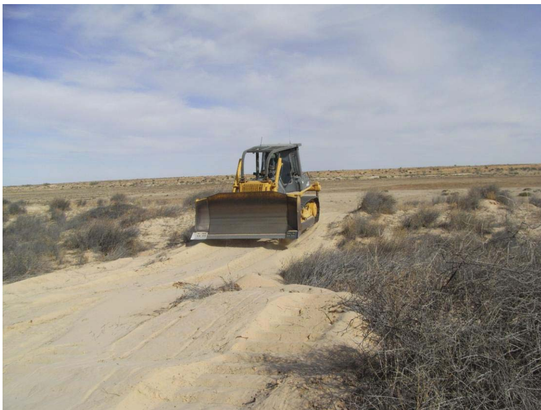
Picture # 7-4: Dozer levelling top of dune.
