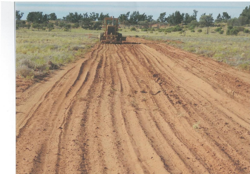
Figure 22: Access track immediately after scarification
