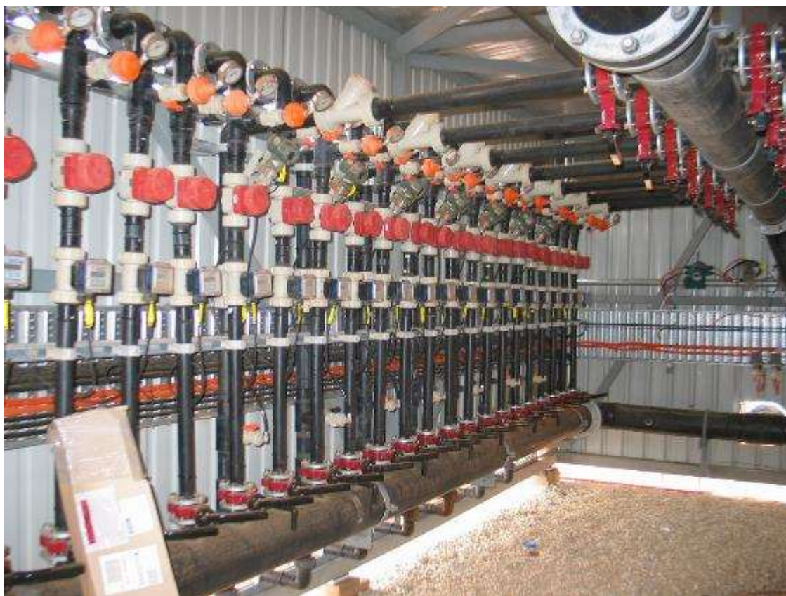
Plate 4-4 Flow Monitoring and Control in a Wellhouse at Pepegoona
