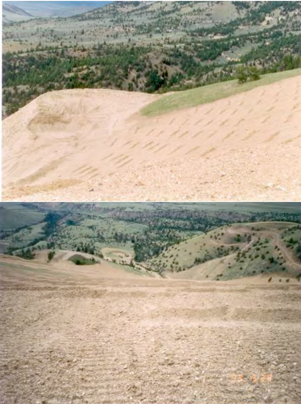
Figure 4 Golden Sunlight Mine (Montana USA). Photos showing re-graded 2H:1V slopes. Lateral Scallop Trenches designed to reduce erosion and rilling. Height of Scallops is approximately 0.5 m and the off-set pattern was designed to slow and retain run-off as it cascades down-slope.
