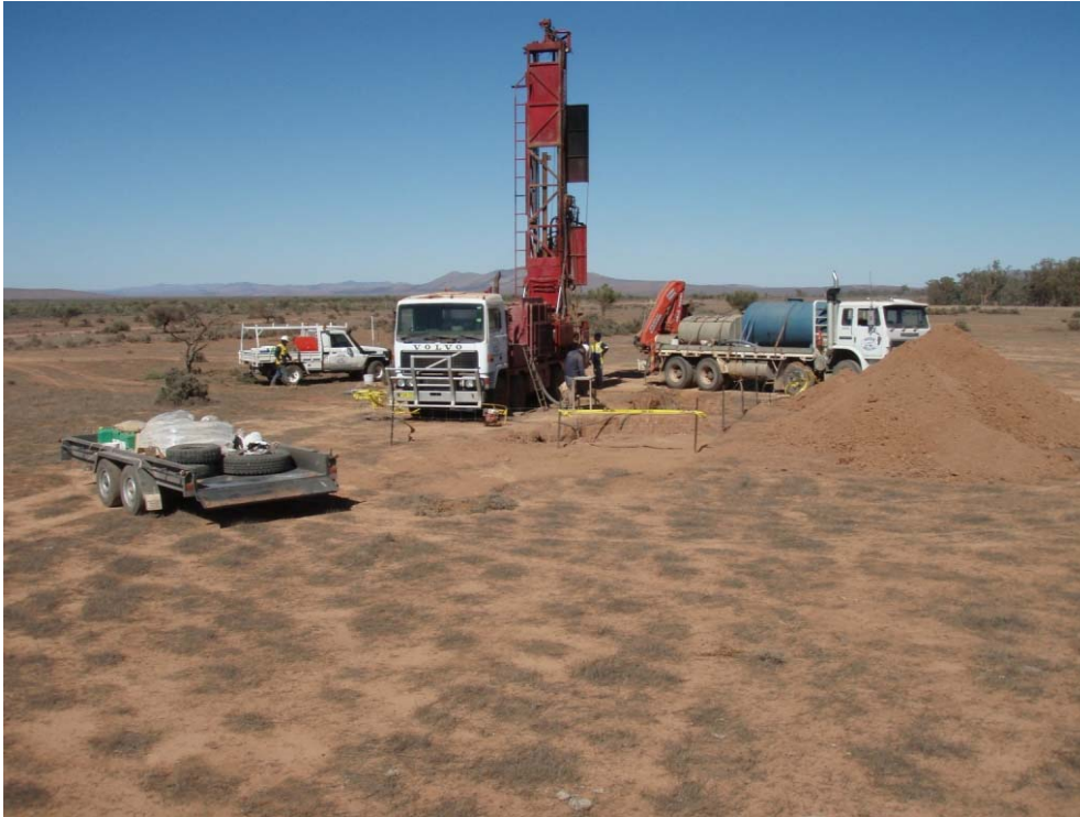
Photo 3 Drill Site FPR H8-1 During Rotary Mud Drilling
