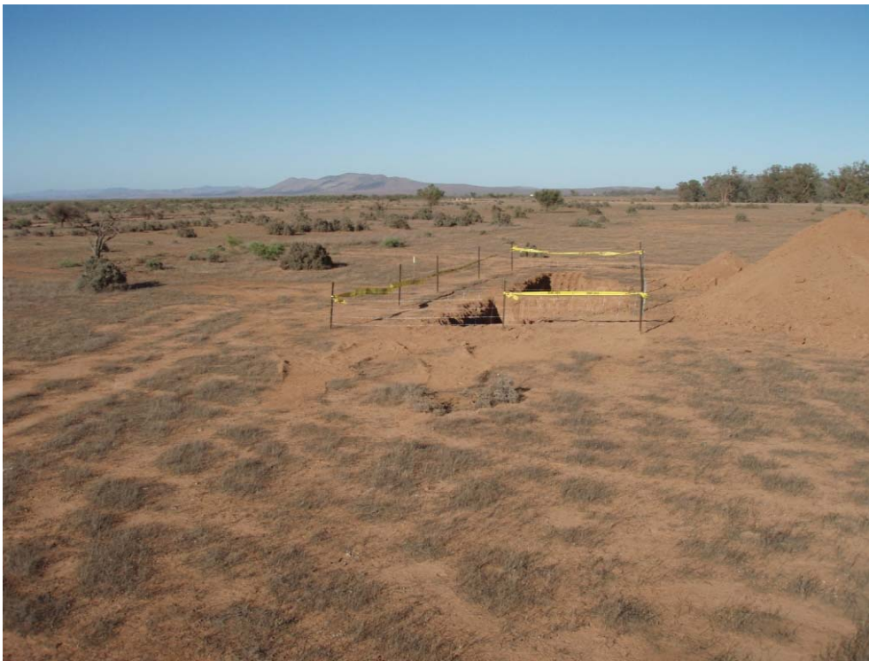
Photo 2 Drill Site FPR H8-1 After mud sump construction
