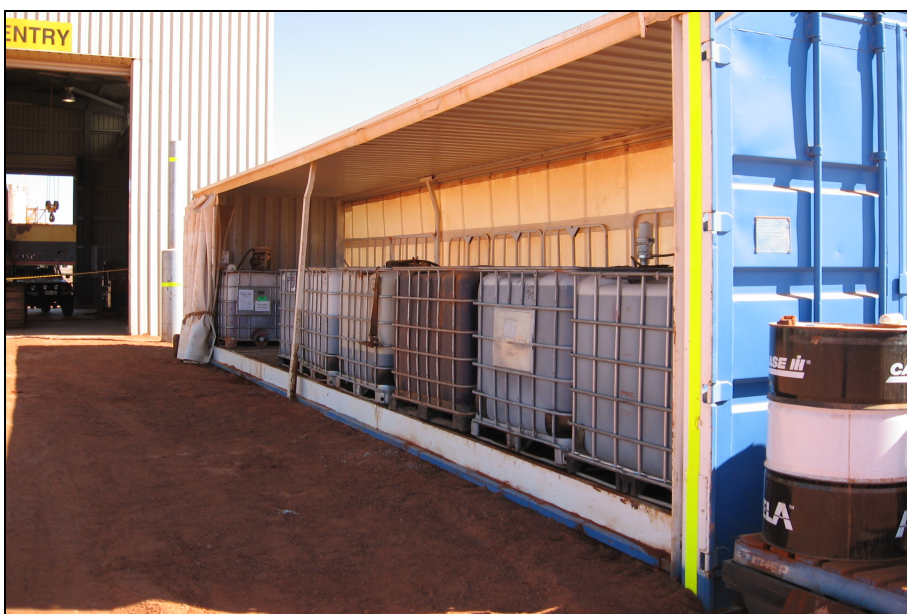
Figure 24: Exact Earthmoving hydrocarbon storage unit.
