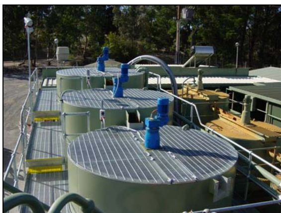
Figure 4: New mixing tanks installed next to the original tanks, doubling the plant's peak treatment capacity.
