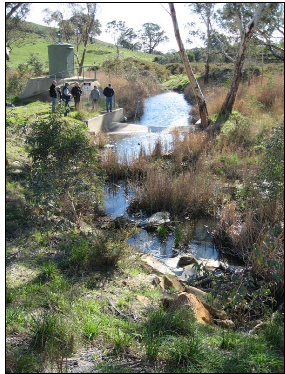
Figure 6: Upstream flat v weir located in Dawesley Creek, for monitoring water flow.
