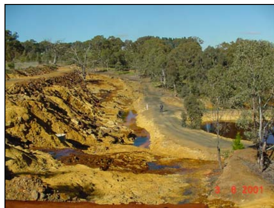
Figure 2. Acid seepage collected at the toe of the wall of the tailings storage facility.
