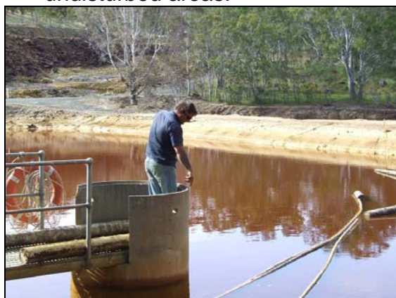
Figure 1. Checking floats and lines on main seepage collection dams.
