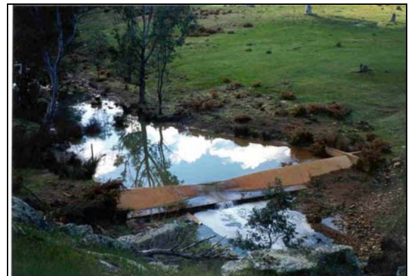
Figure 7: Downstream v weir monitors the volume of water leaving the site.
