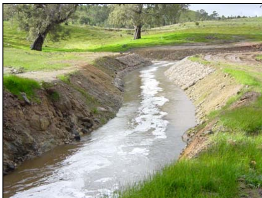
Figure 3: Open section of the diversion drain carrying Dawesley Creek flow past the mine
