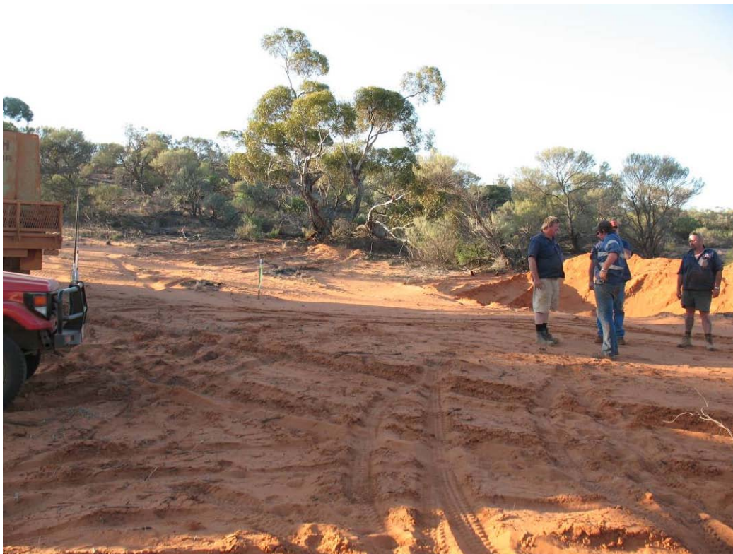
Figure 2: Drillsite YDRC001 prepared drill site prior to drilling (looking northeast) – 09/2008
