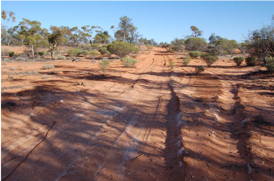
Photo 15: Multiple tracks and widening along northern access track to drill sites. Track width had not been kept to a minimum.
