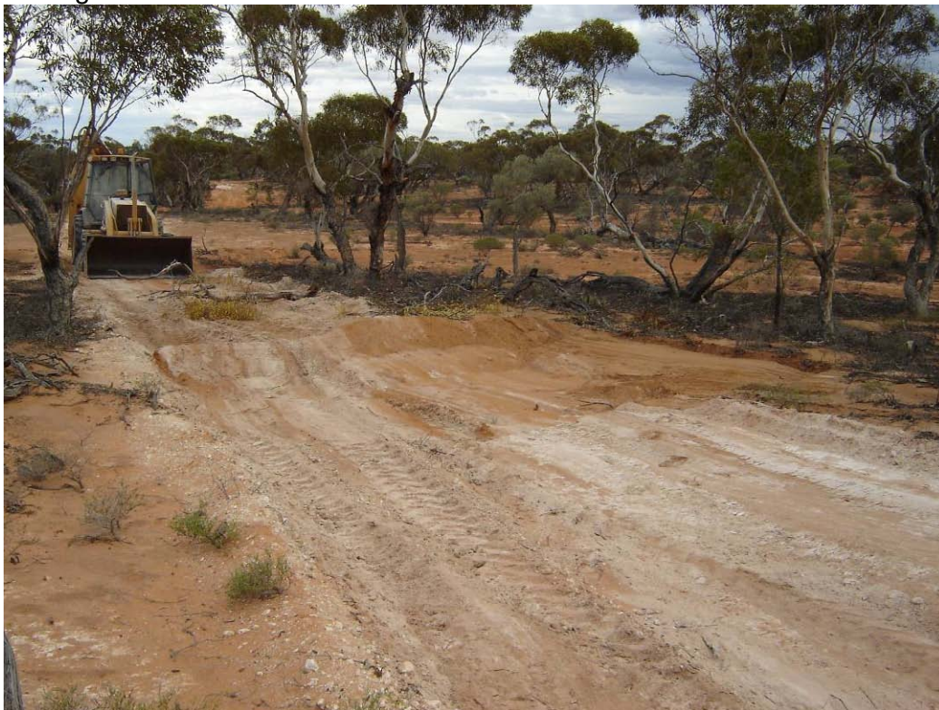
Figure 8: Rehabilitation of access track at approx coordinate 440600E/6572000. The rehabilitation here shows a small "run-off check" on a
