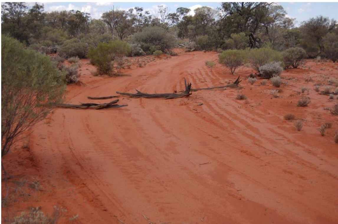
Photo 5: Same as photo 2 where portion of track has been previously ripped and branches have been recently placed across the track.
