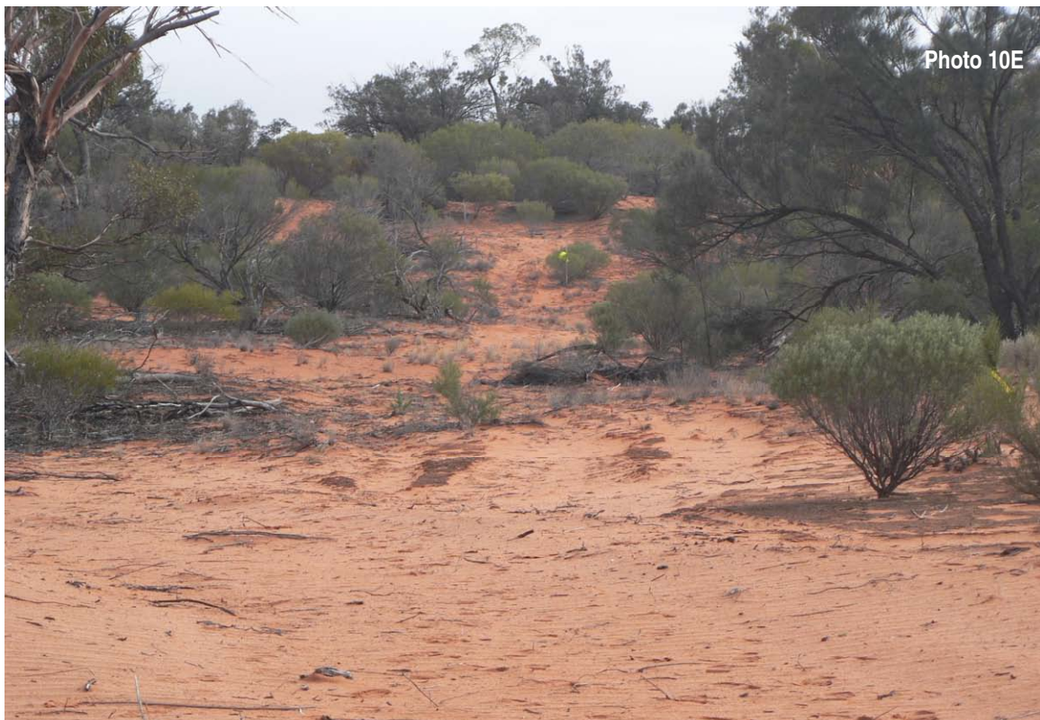
PHOTO PLATE 10 WGS 84 June 2009 Location: 441550 mE 6570130 mN Photo 10E and 10F: Looking north, 60 mt north of the entrance in Photo10A/B at the first attempted dune crossing. Wheel tracks have been lifted and raked, windrows where obvious have been levelled with vegetation spread around to close in the open area
