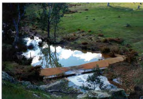
Fig 7. Downstream v-notch weir monitors the volume of water leaving the site.
