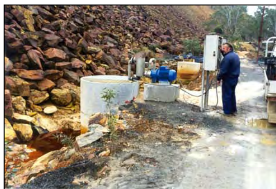
Fig 1. Collecting acid seepage at the toe of the southern waste rock dump.
