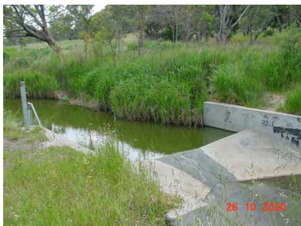
Fig 6. Upstream v-notch weir located in Dawesley Creek, for monitoring water flow.
