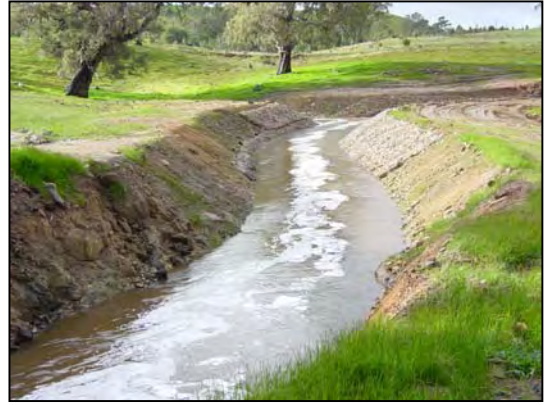
Fig 3. Open section of the diversion drain carrying Dawesley Creek flow past the mine
