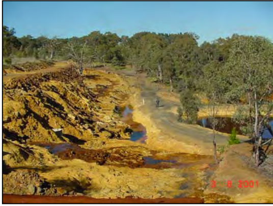
Fig 2. Acid seepage collected at the toe of the wall of the tailings storage facility.
