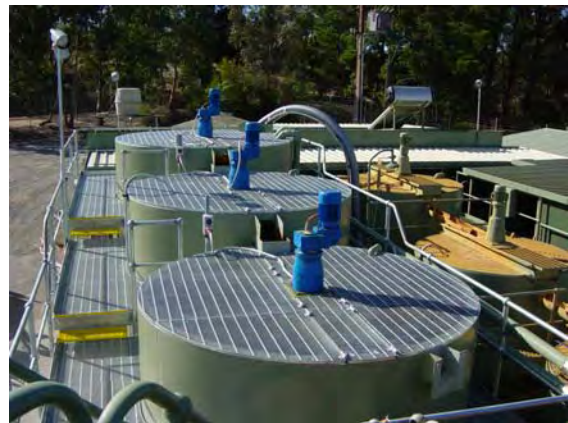
Fig 4. New mixing tanks installed next to the original tanks, doubling the plant's peak treatment capacity.
