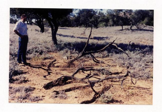
PLATE 2: Rehabilitation near trenches THT-3 (foreground) and THT-4 (RHS of photograph, background). Methods employed to minimise erosion have succeeded. Photograph taken approximately 14 months after excavation of trenches.
