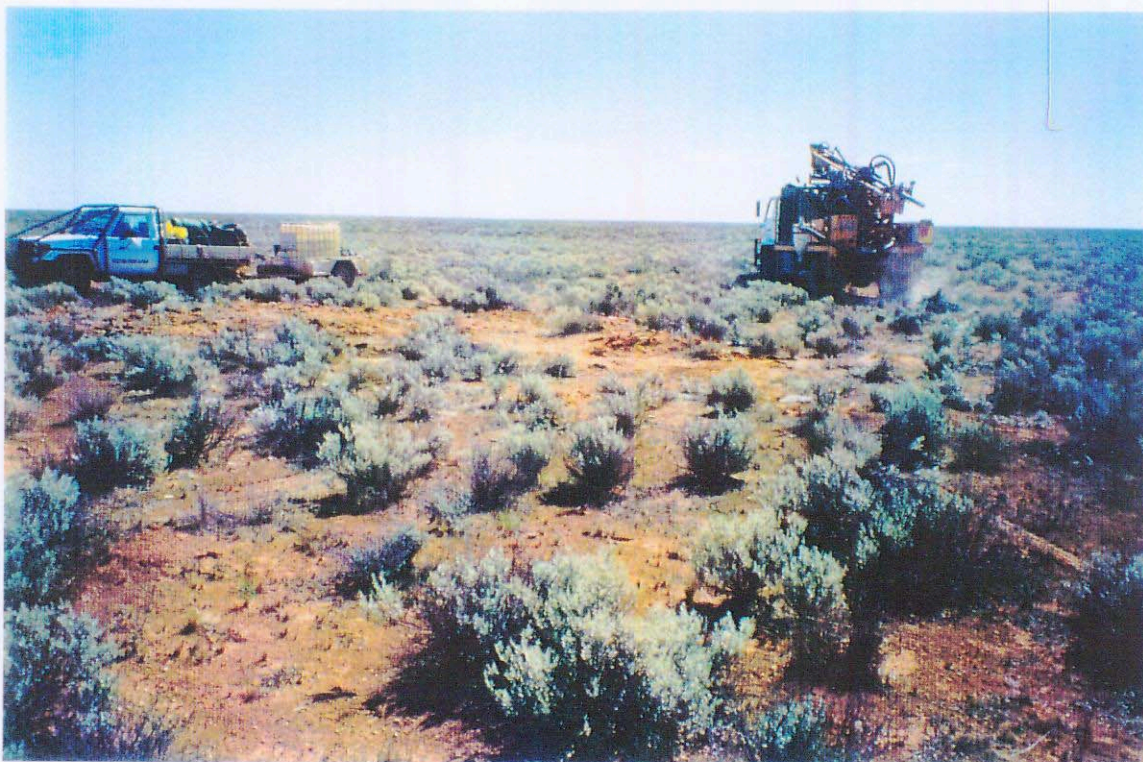
Plate 8: Drillsite at OS-4 prospect after backfilling and cleanup. Drill rig has moved off drillsite and sample pits were located on left of photo.
