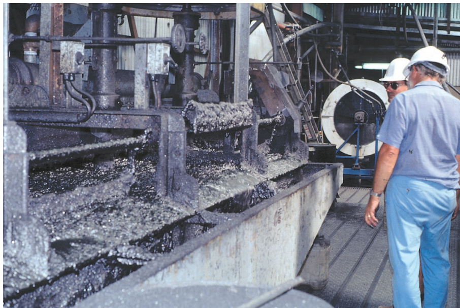
Graphite concentrate being collected from flotation cells at the Uley Mine, February 1993. (Photo 47522)
