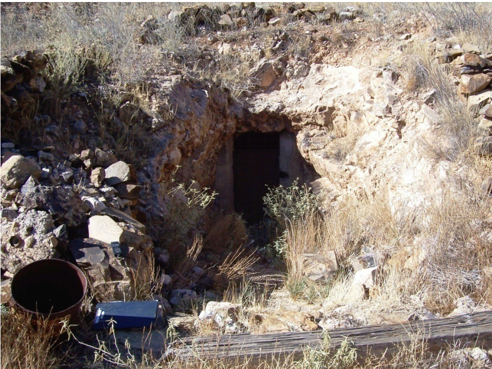
Plate 37. Adit B2, entrance to Takati Mine, 2016.
