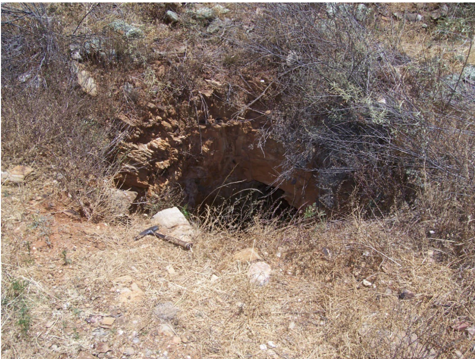
Plate 29. Adit 13, entrance to Golden Harp Mine, south adit (b).
