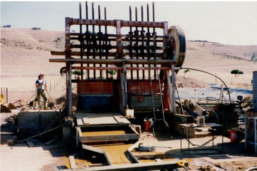
Plate 4. Rebuilding of battery by lease holder Kevin Wallace, with 5 stamps operating, 1993. (Photo 041482)
