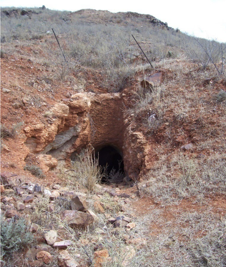
Plate 32. Entrance to Central Mine Adit 2 with vertical shaft above.
