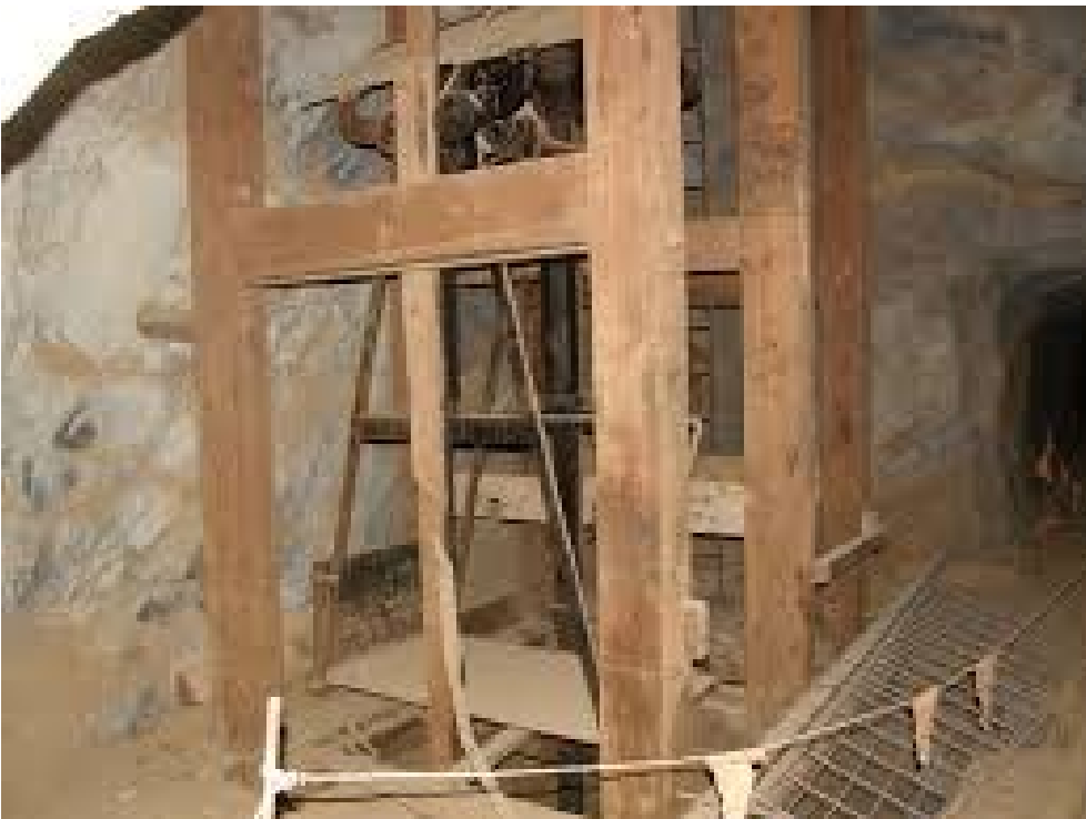
Plate 21. Byles Mine three compartment internal shaft, main adit, 28 m level.
