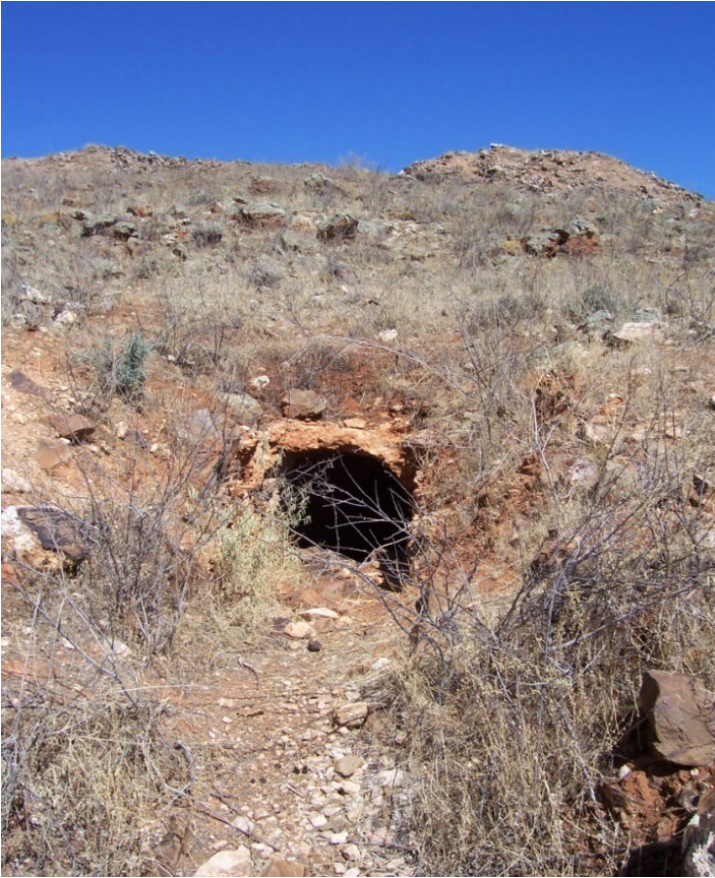
Plate 42. Adit A7, entrance to adit, Cox Sandstone above.
