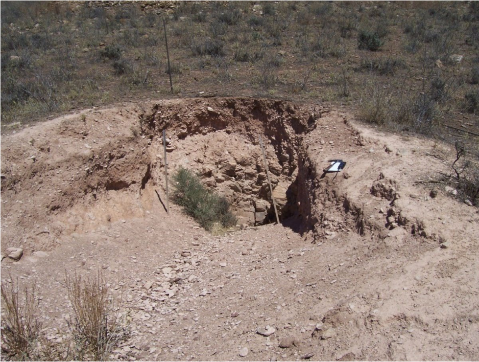
Plate 14. Adit 1, Hansel & Mundy Mine, adit entrance collapsed.
