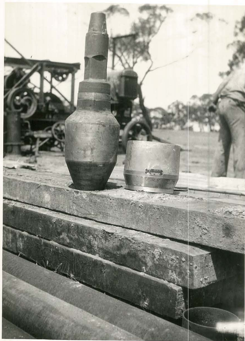
Bordertown Bore. Screen Top and Expanding Tool.
