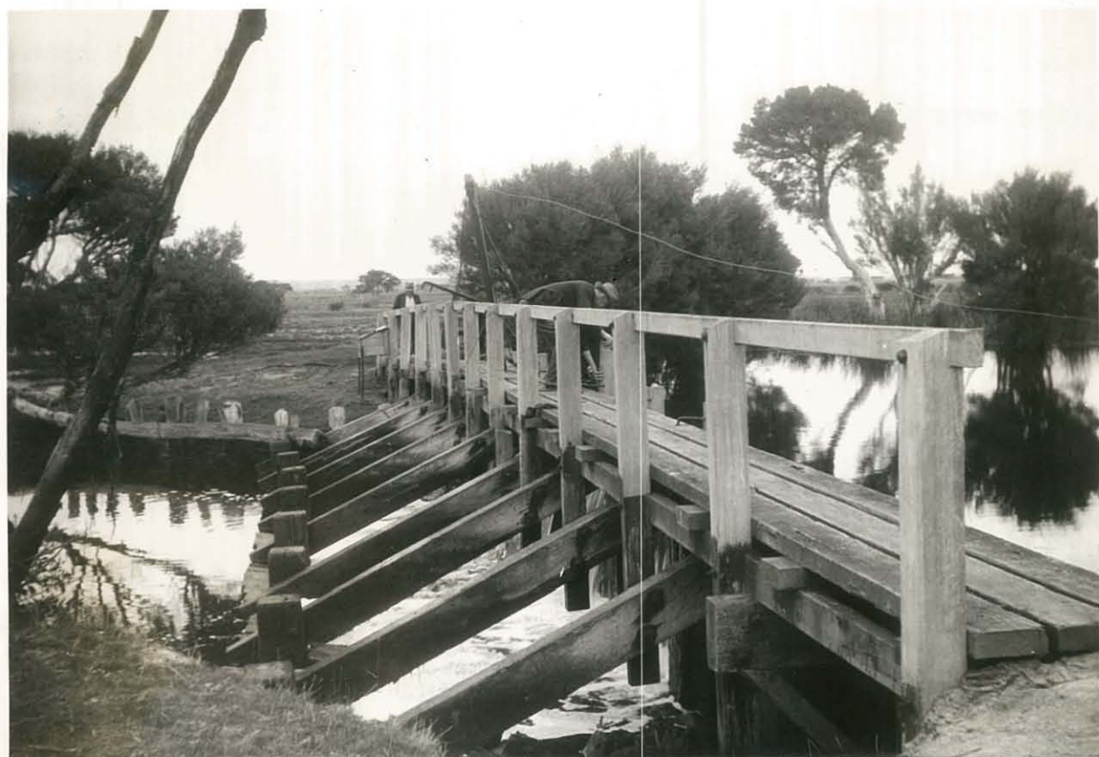
Timber Barrage at Kingscote.
