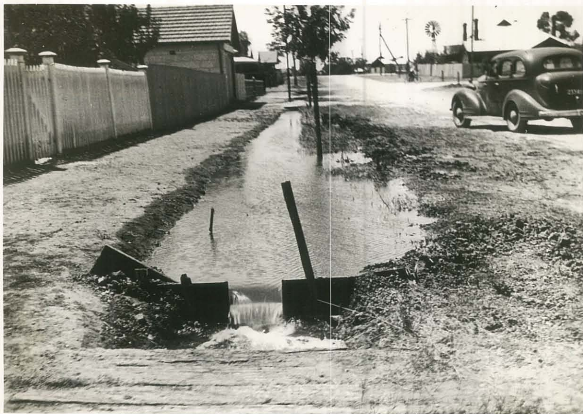
Bordertown Bore. Test Measuring Weir.
