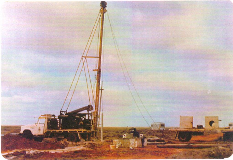
Plate 1. Cable tool rig on site. Slide No. 13133
