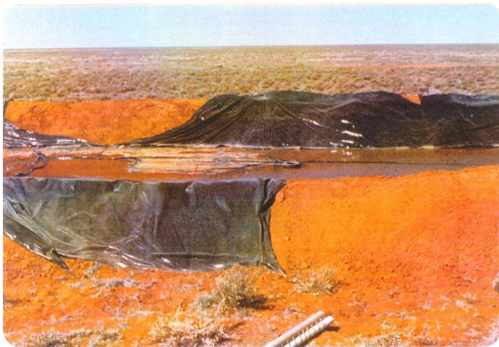
Plate 4. Storage dam showing wind damage to plastic lining. Slide No. 13230.
