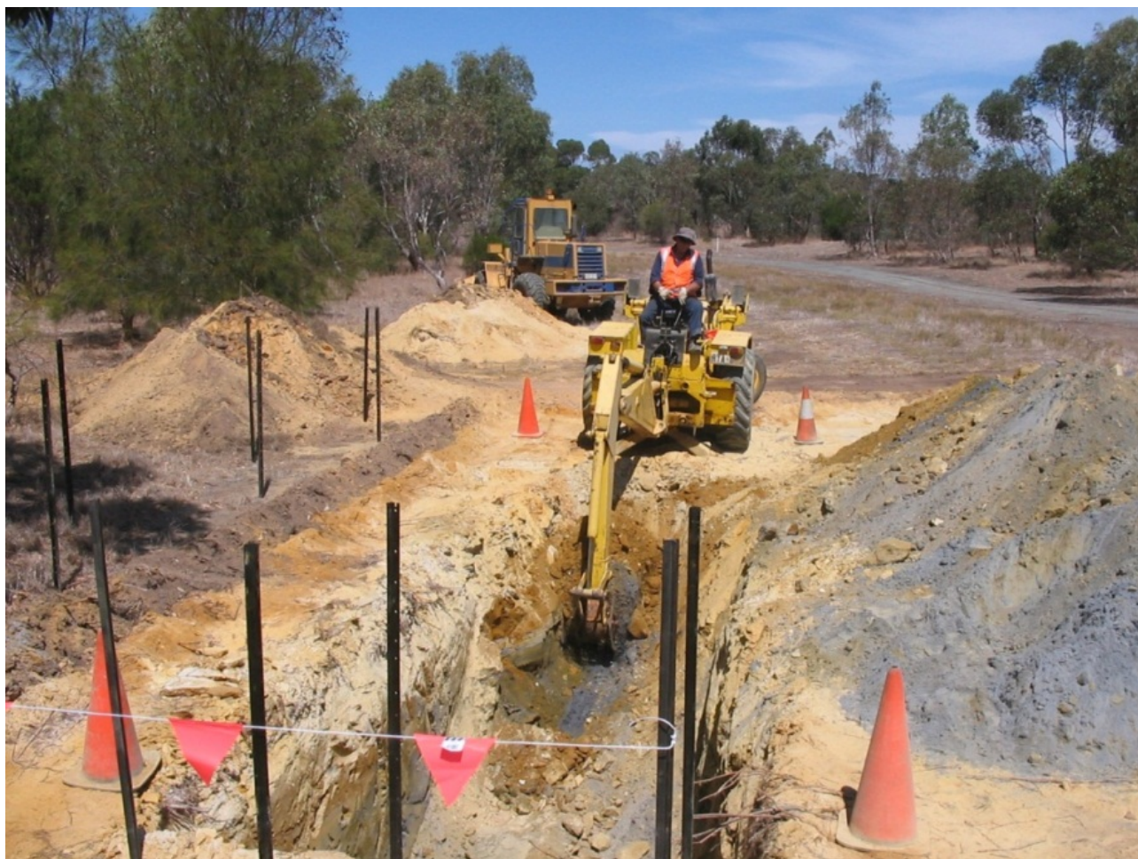
Figure 2. Excavation of tailings in February 2012 showing pale yellow brown oxidised tailings and grey un-oxidised materials below 1 m depth. (Photo 414503)
