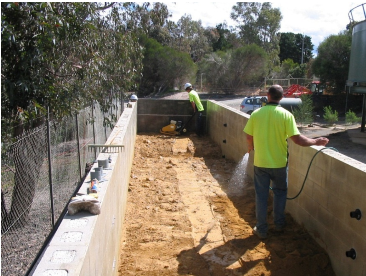
Figure 13. Wetting up and compacting the PAF mix within the geochemical test-cell. (Photo 414514)
