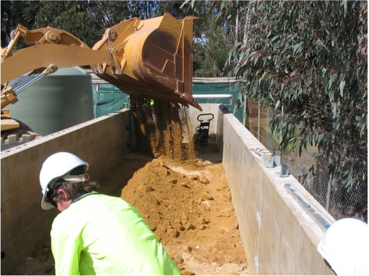
Figure 12. Dumping PAF mix into the geochemical test-shell, composed of besser blocks. (Photo 414513)
