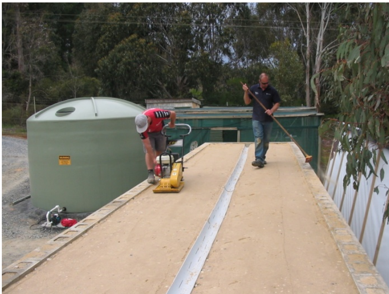
Figure 15. NAF cover surface with gutter to simulate a creek-line (note: 23 kL water storage tank on left and cover lid frame to the right). (Photo 414516)
