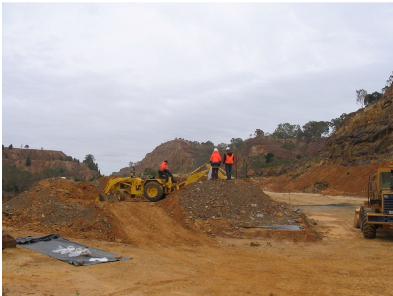
Figure 3. Excavation of waste rock from Pyramid #3 with collection of sub-samples for sulfur speciation testwork. (Photo 414504)
