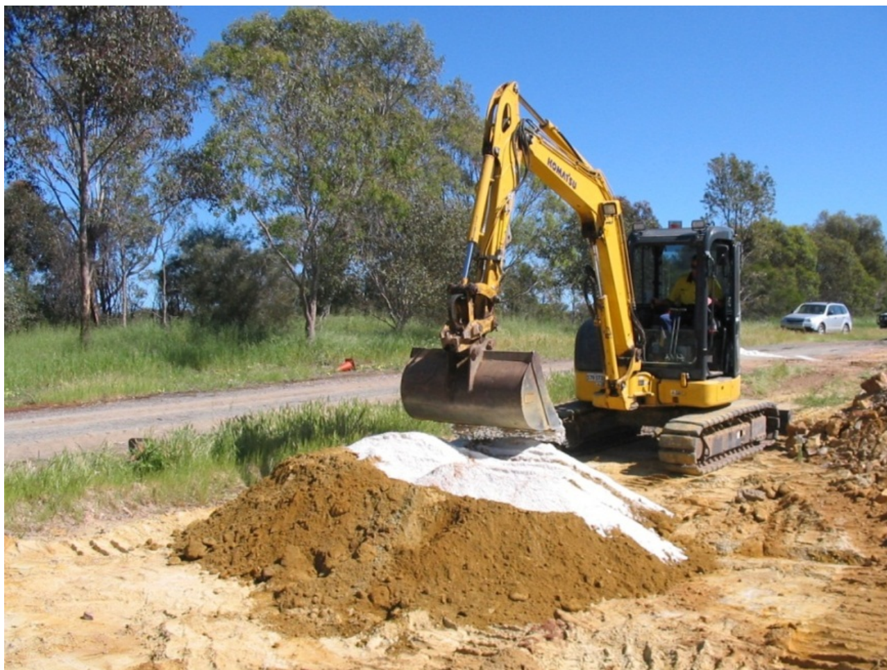
Figure 11. Mixing waste rock, tailings and lime for 100 t presentation trial. (Photo 414512)
