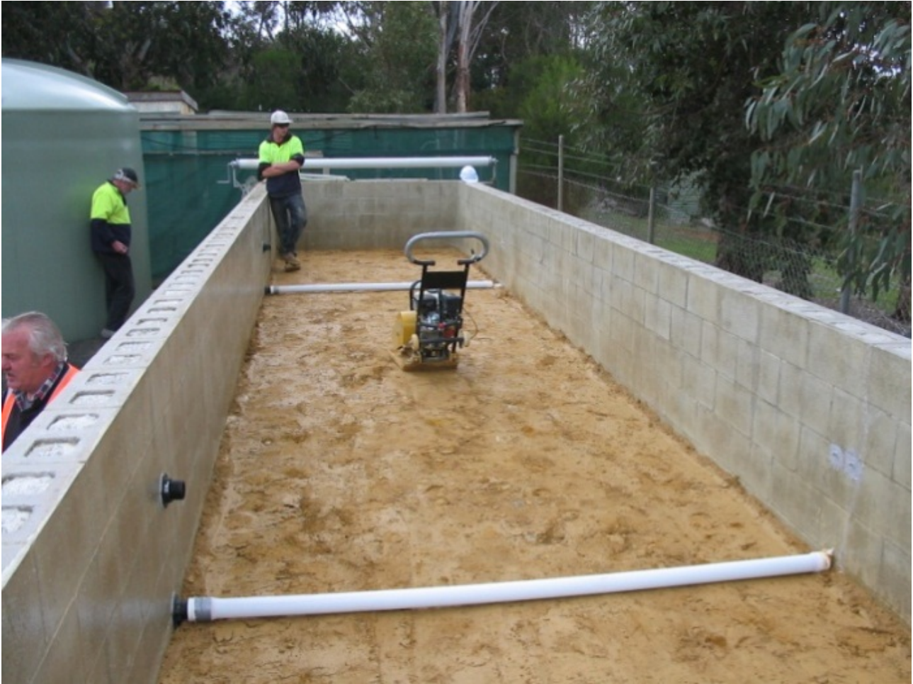
Figure 14. Piezometers placed horizontally across the width of the test-cell. (Photo 414515)
