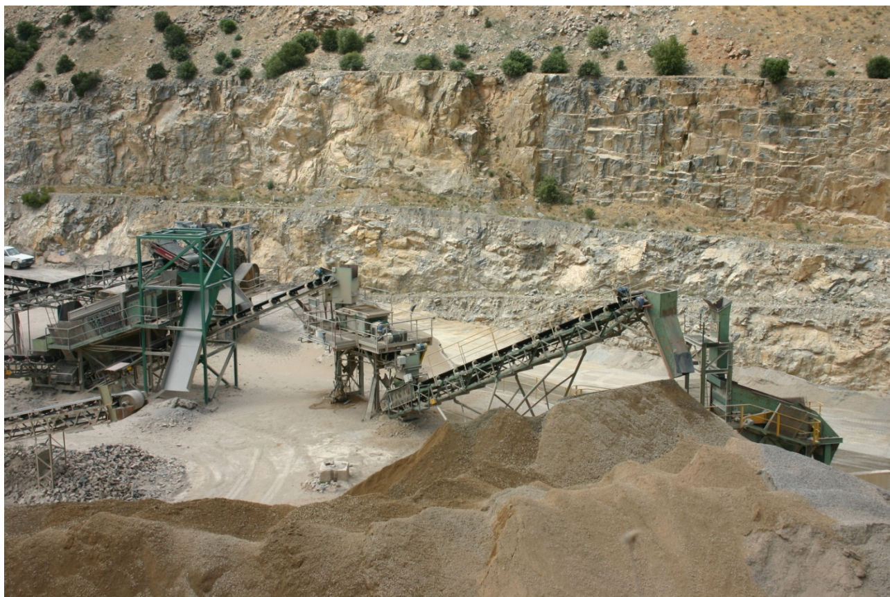
Sellicks Hill quarry and crushing plant. (Photo 408652)
