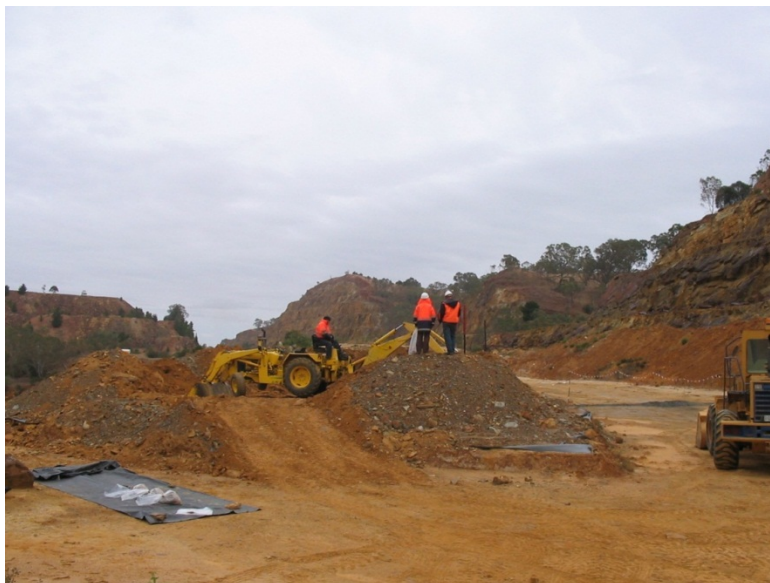
Figure 3. Excavation of waste rock from Pyramid #3 with collection of sub-samples for sulfur speciation testwork.
