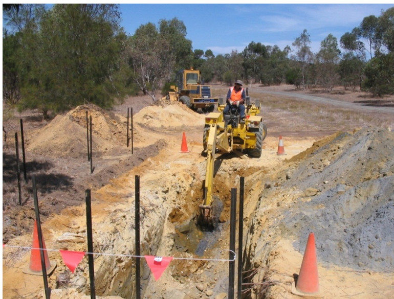
Figure 2. Excavation of tailings in February 2012 showing pale yellow brown oxidized tailings and grey un-oxidized materials below 1 m depth.
