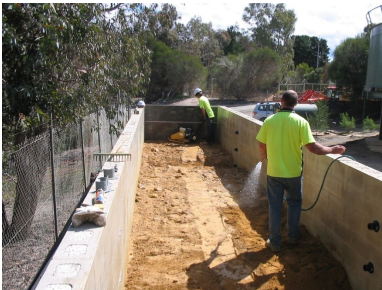
Figure 13. Wetting up and compacting the PAF mix within the geochemical test-cell.
