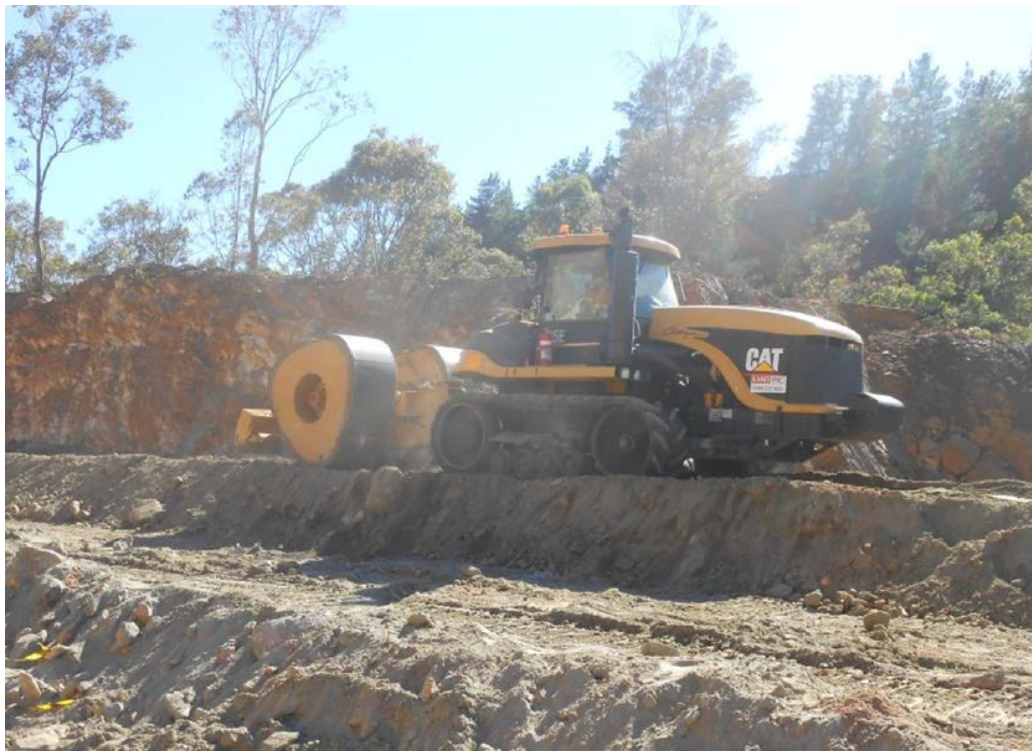
Figure 12. Impact Roller at Phase 3 trial embankment.
