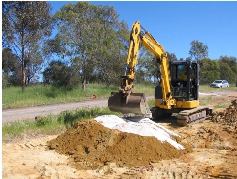
Figure 11. Mixing waste rock, tailings and lime for 100t presentation trial.
