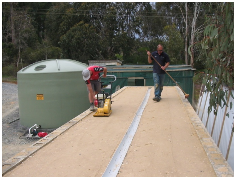
Figure 15. NAF cover surface with gutter to simulate a creek-line (note: 23kL water storage tank on left and cover lid frame to the right).
