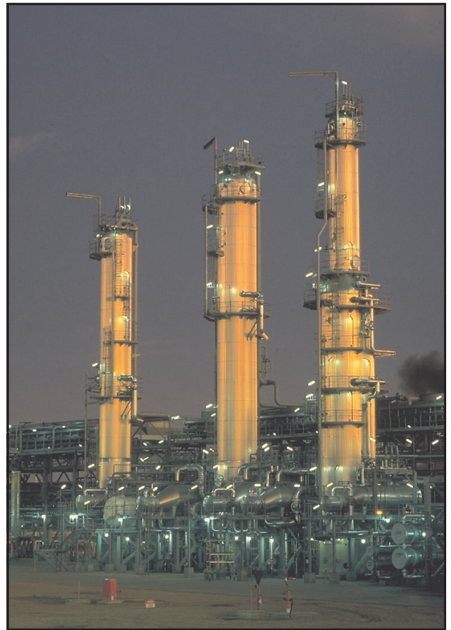
Fractionation plant at night, Port Bonython, July 1984. (Photo 43378)
