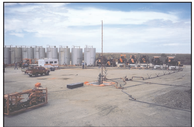
Surface equipment used during hydraulic fracturing, Tirrawarra 48. (Photo 45948)
