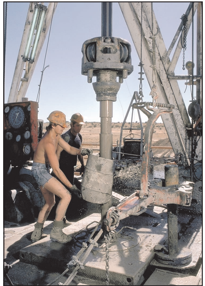
Drilling, Toolachee Field 1984. (Photo 43367)
