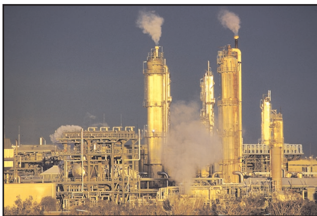
Carbon dioxide removal towers, Moomba. (Photo 43373)
