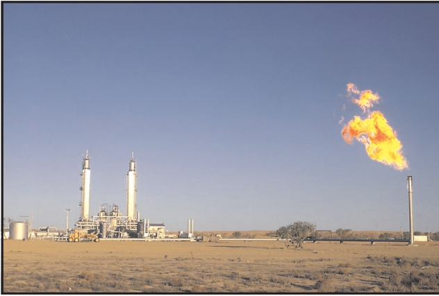
The Moomba Natural Gas Processing Plant in November 1969. (Photo 43830)
