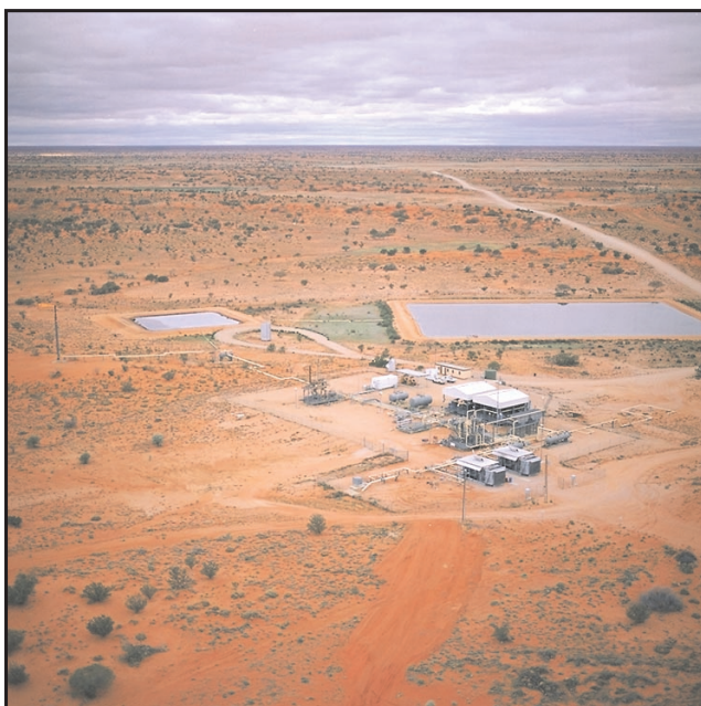
Cooper Basin satellite facilities. (Photo 43790)
