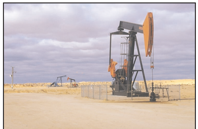
Beam pumps producing oil, Merrimelia Field. (Photo 45016)
