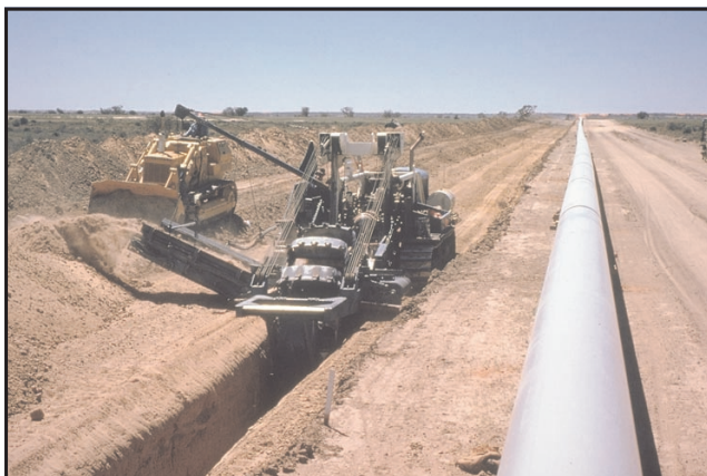
Construction of Della trunkline. (Photo T15557)
