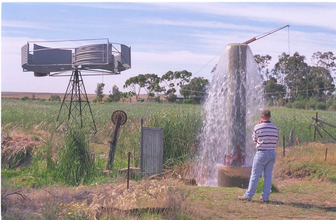
Overflow of excess water from a main supply channel
