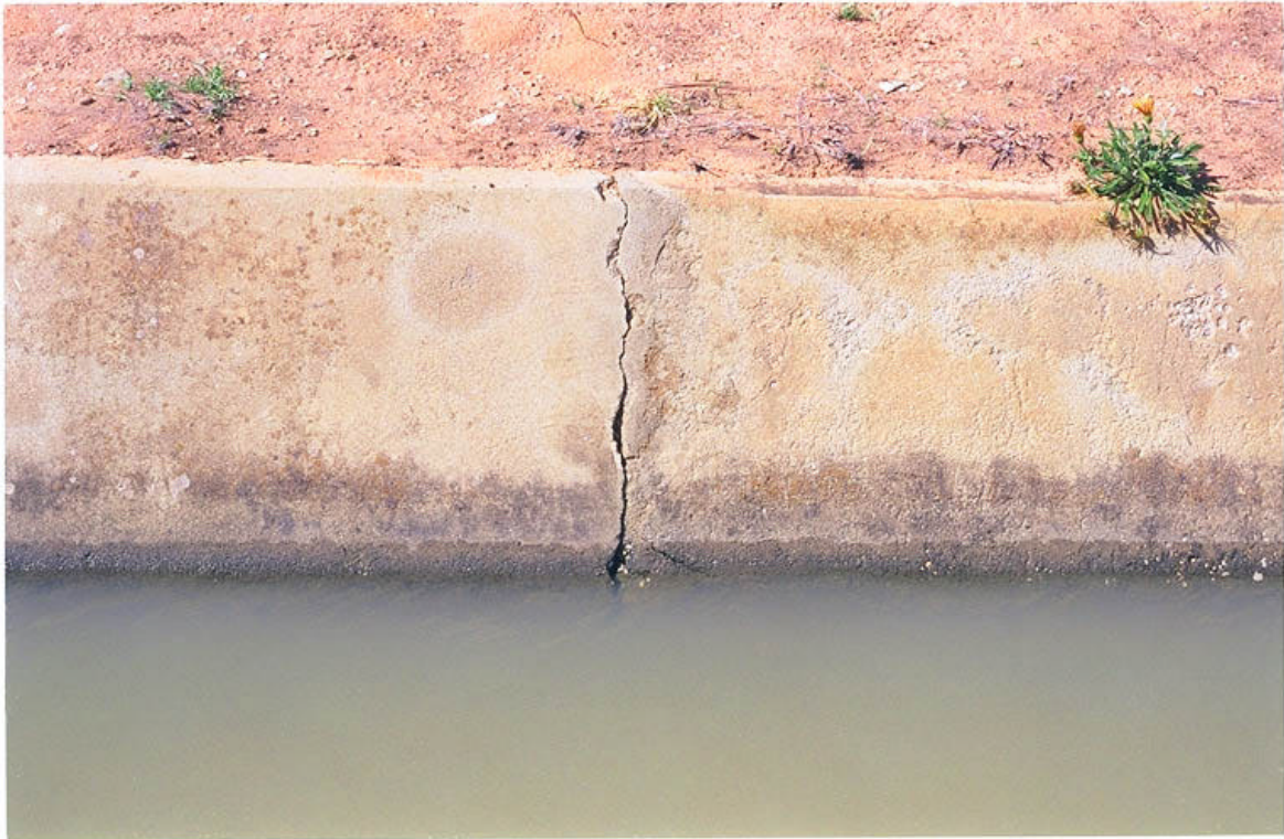
Cracks in the delivery channel which allow seepage
